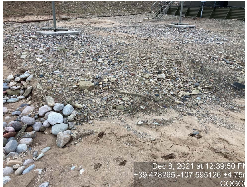
Erosion/sediment migration/failing BMP
