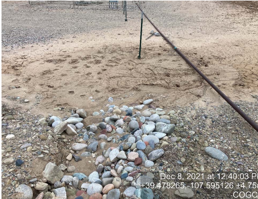
Erosion/sediment migration/failing BMP
