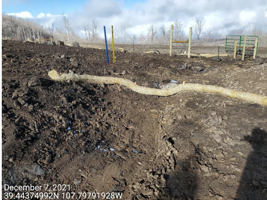
Photo 6: Photos provide example of straw wattles observed implemented on the west end of the Location. Photos show wattles have not been installed per good engineering practices; wattles have been placed/staked upon the surface, and have not been trenched and backfilled.
