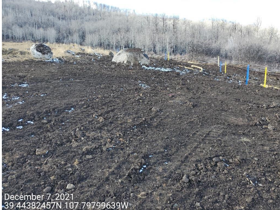
Photo 5: Photos examples showing the recently disturbed areas along the west end of the Location; re-seeding evident. Photos show stormwater and erosion control measures to stabilize soils are missing or insufficient.
