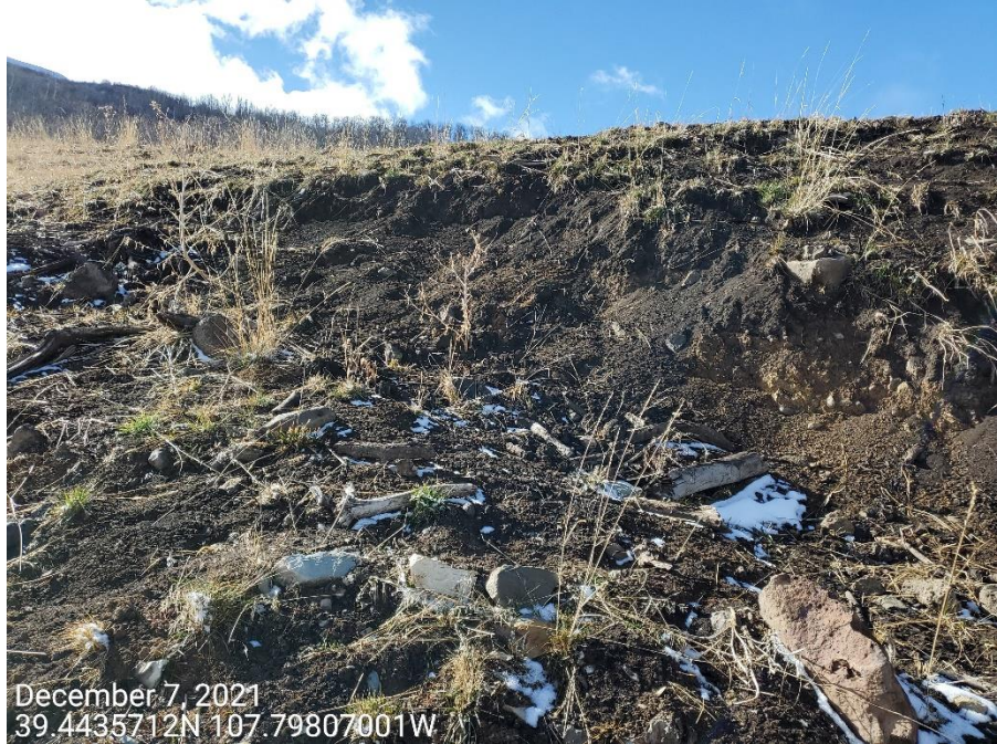
Photo 4: Photos examples showing control measures to protect and stabilize the cut slopes of the Location are missing or insufficient; erosion degradation evident.
