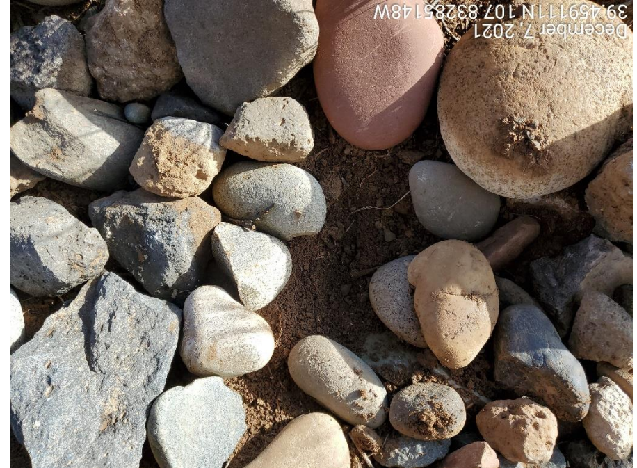
Photo 2: Photo shows Operator has constructed a shallow sediment trap at the end of the ditch; outlet missing geotextile lining beneath the rip-rap material per good engineering practices.
