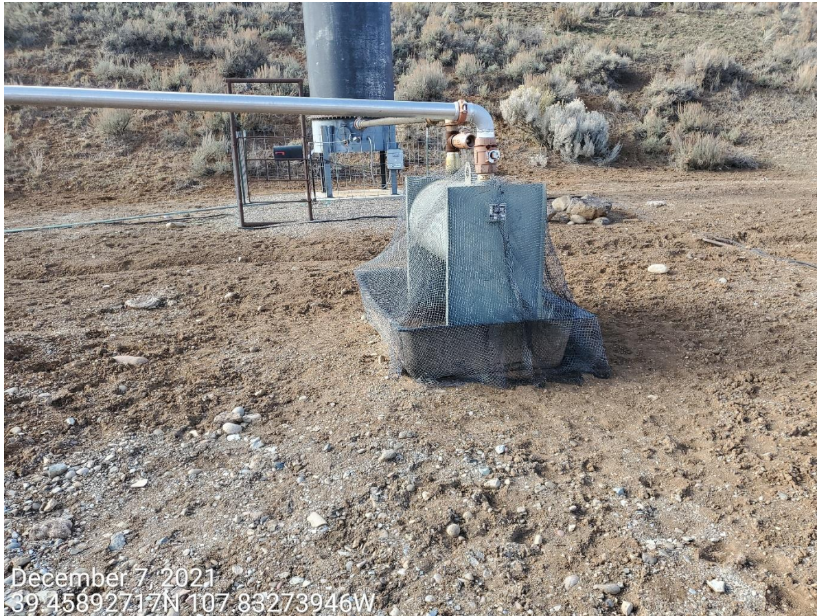
Photo 3: Photo shows controls measures (netting) has been implemented at the containment BMP to prevent wildlife .
