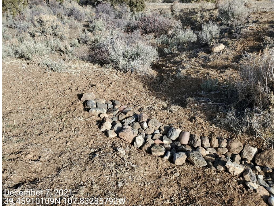
Photo 2: Photo shows Operator has constructed a shallow sediment trap at the end of the ditch; outlet missing geotextile lining beneath the rip-rap material per good engineering practices.
