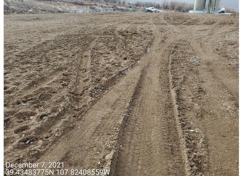
Photo 4: Photos taken from the production areas of the Location. Photos provide examples showing that control measures to stabilize the production areas, and to mitigate tracking and offsite sediment transport remain missing or insufficient.
