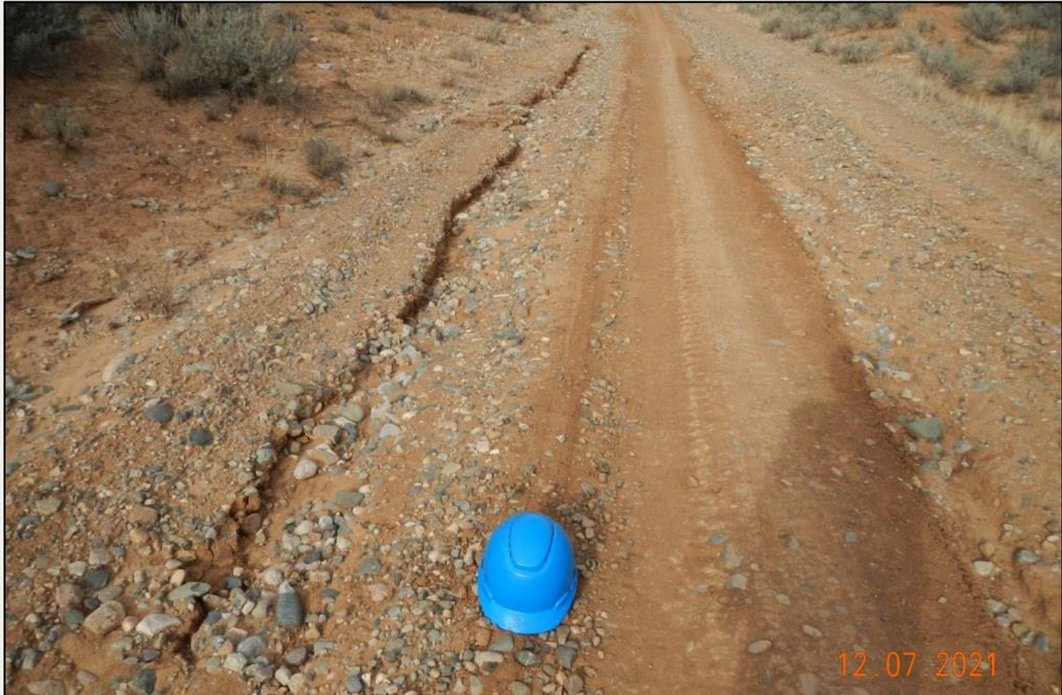
Photo 4. View of erosional channeling occurring on the access road, approximately 6-12 inches wide and deep. Road needs long-term stabilization. Hard hat in place for scale.
