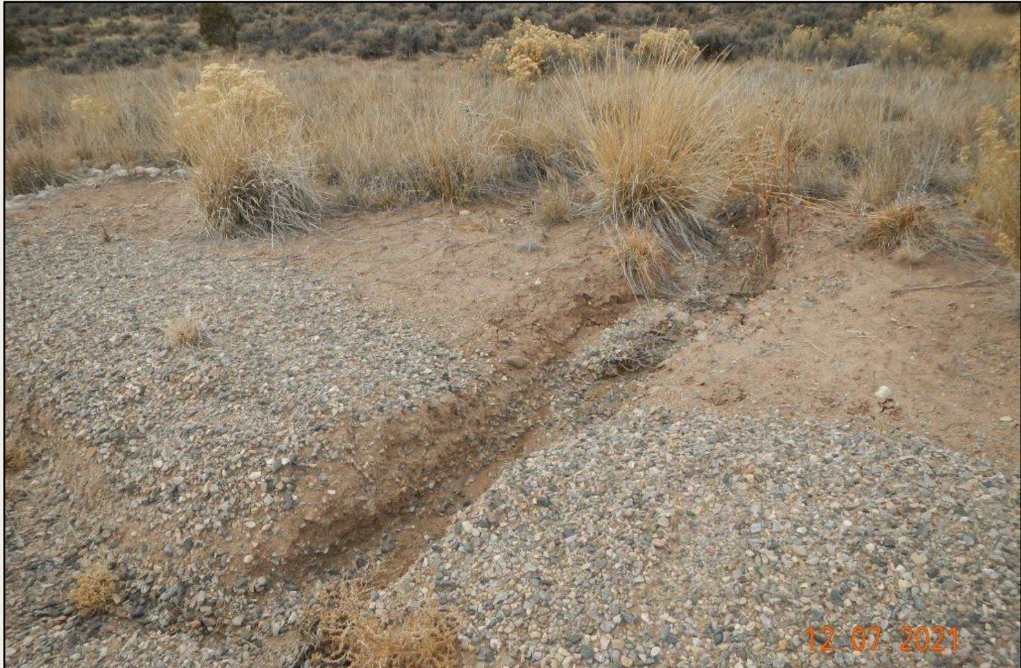
Photo 4. View of an erosional channel approximately 1ft wide and deep, within the northern project area, needing stabilization.
