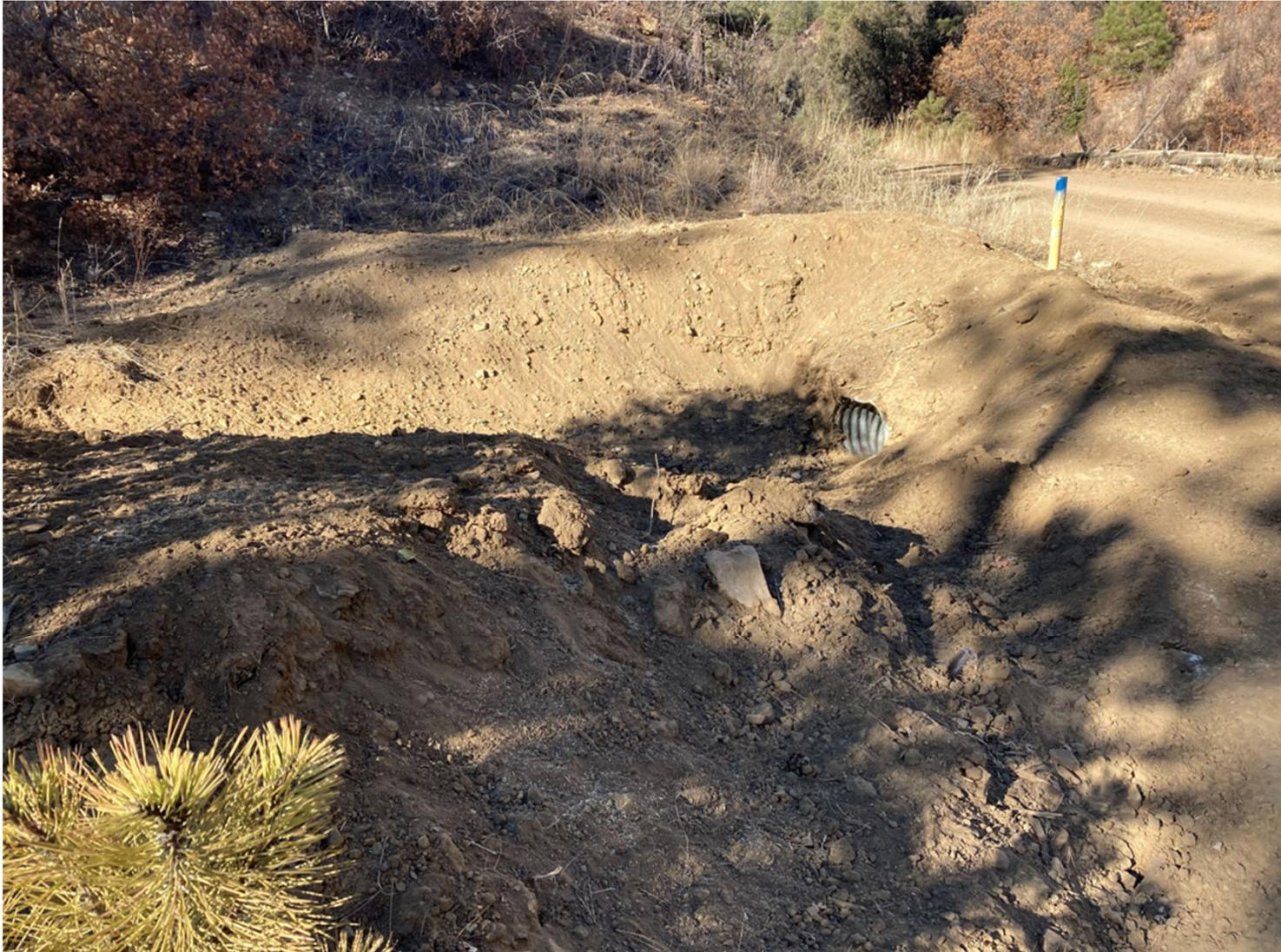
THE DIRT BERM PLACED AROUND THE CULVERT INLET WAS SEEDED WITH AN APPROVED CPW SEED MIX TO PROMOTE THE ESTABLISHMENT OF VEGETATION.
