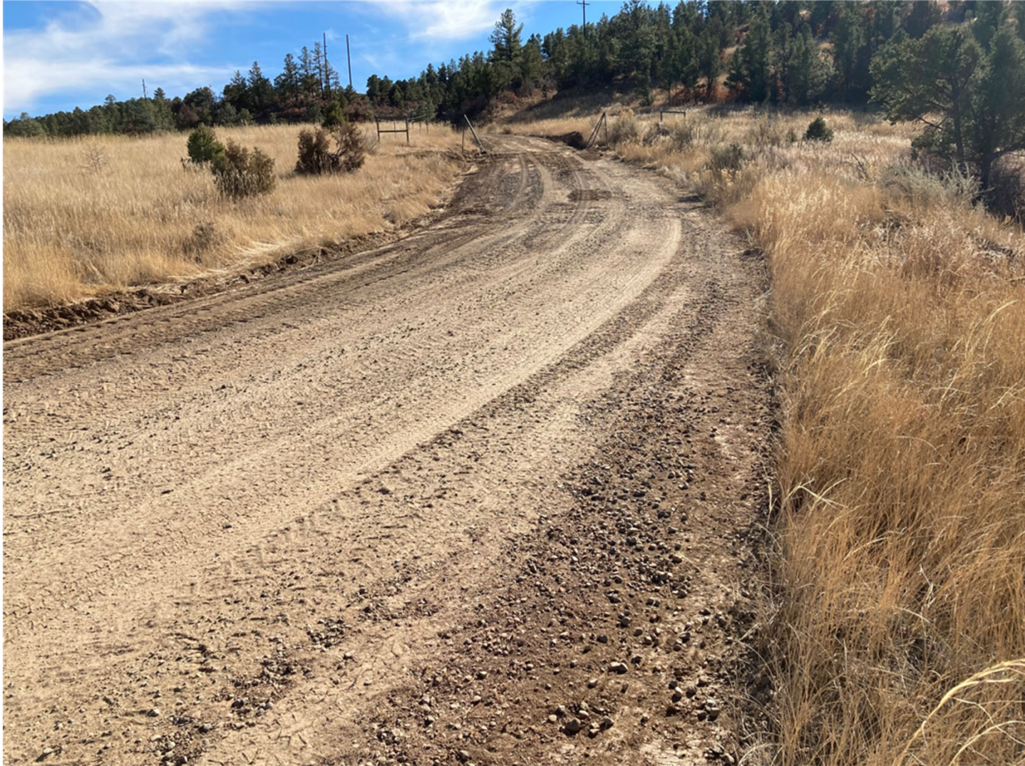
THE MAIN LEASE ROAD WAS SURFACED CROWNED TO CORRECT THE SURFACE EROSION AND CREATE SHEET FLOW.
