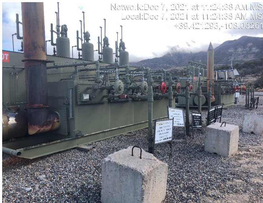
Photo #5332 Multiple unmarked storage tanks.
