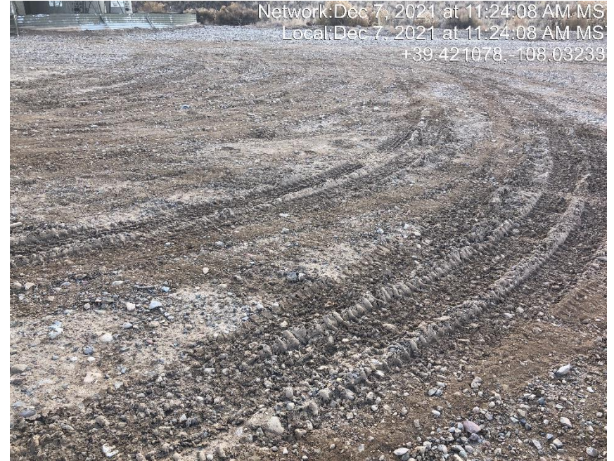
Photo #5331 Location lacks stabilization.
