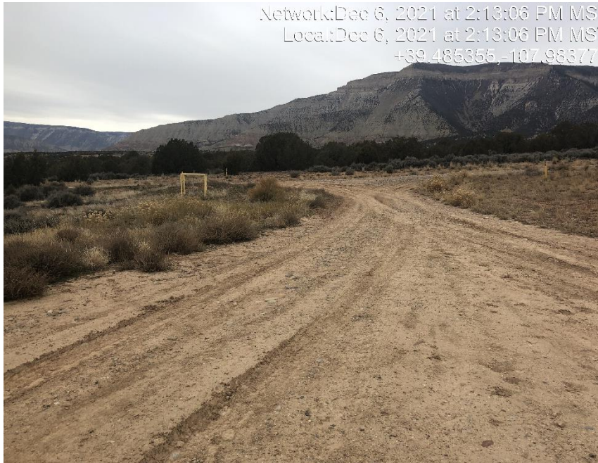
Photo #5325 Insufficient Tracking BMP at entrance to location.
