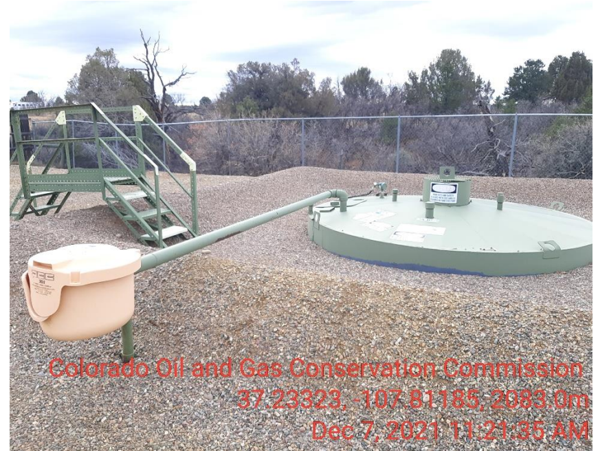
Photo 4 produced water tank
