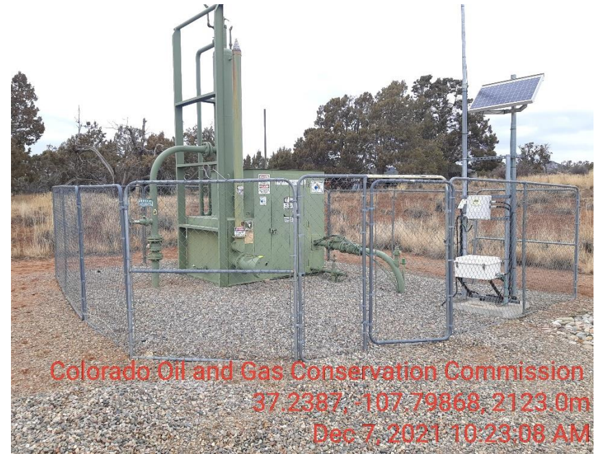
Photo 4 Vert Sep and meter run
