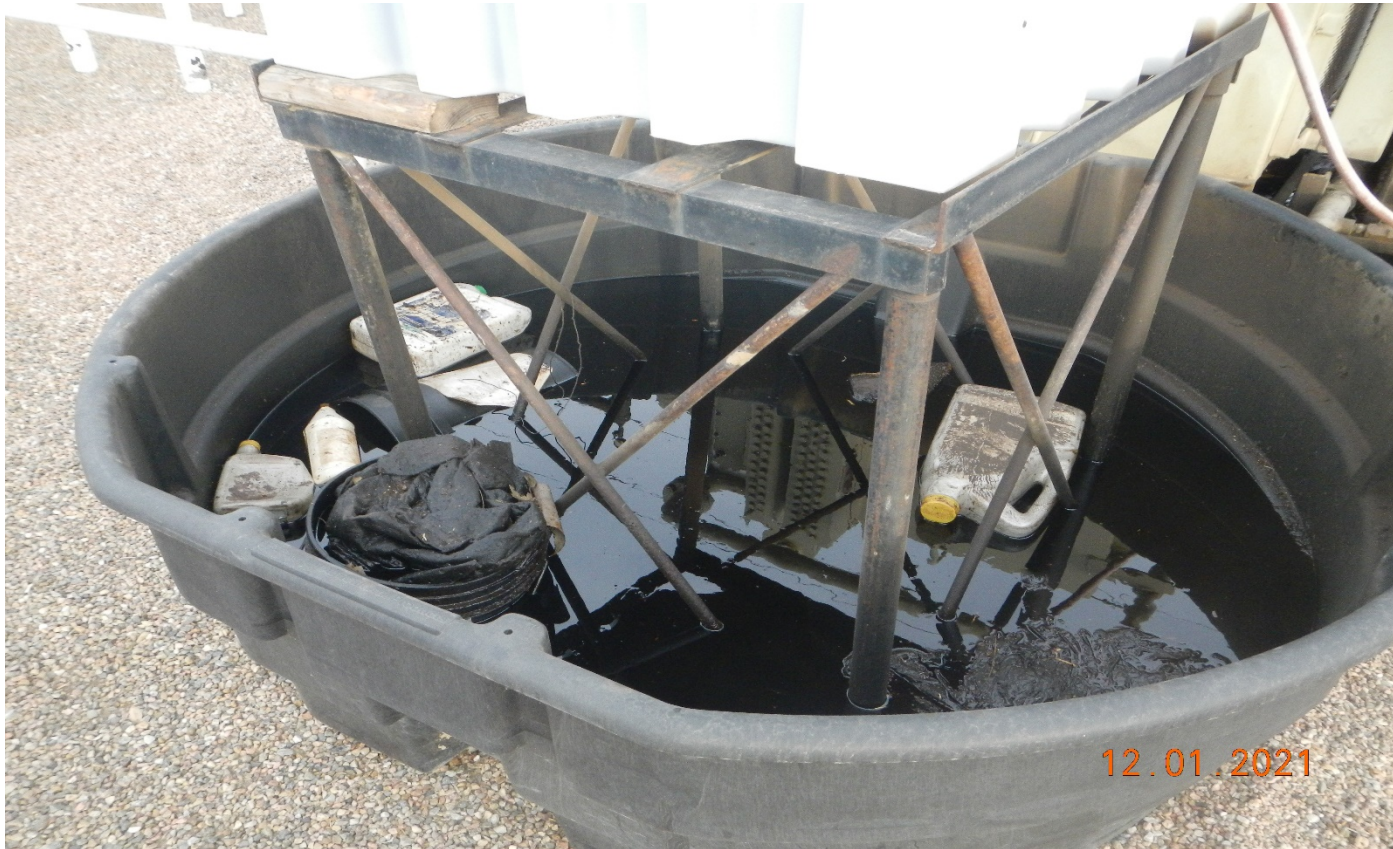
Photo 3. There is oil and trash inside the secondary containment. This needs to be cleaned up and properly disposed.
