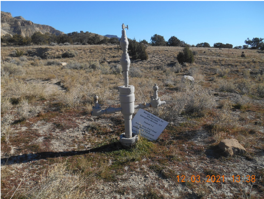
Wellhead with sign. Temporarily abandoned.
