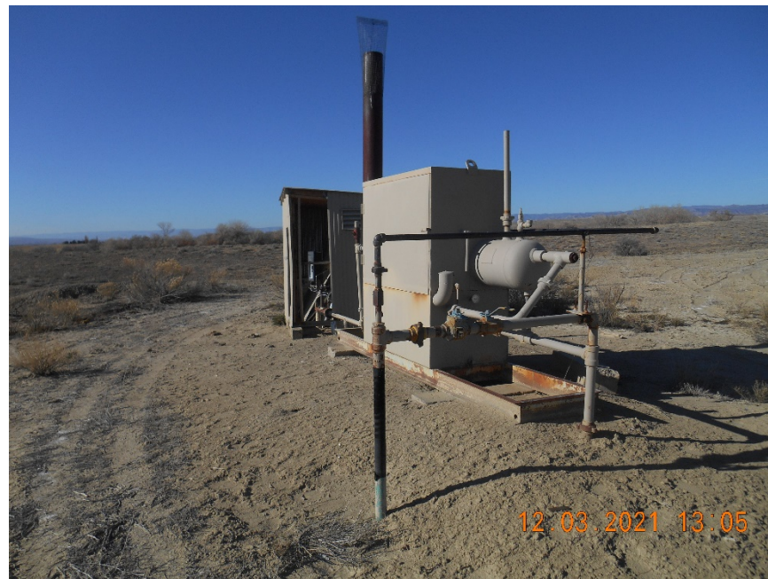
Separator and Meter housing
