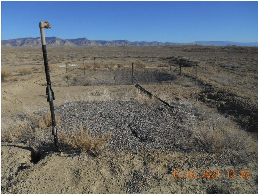
Blowdown pit with fence and netting. Tank removed. Unused 2" riser and pipe.
