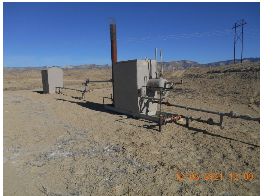
Separator and Meter housing
