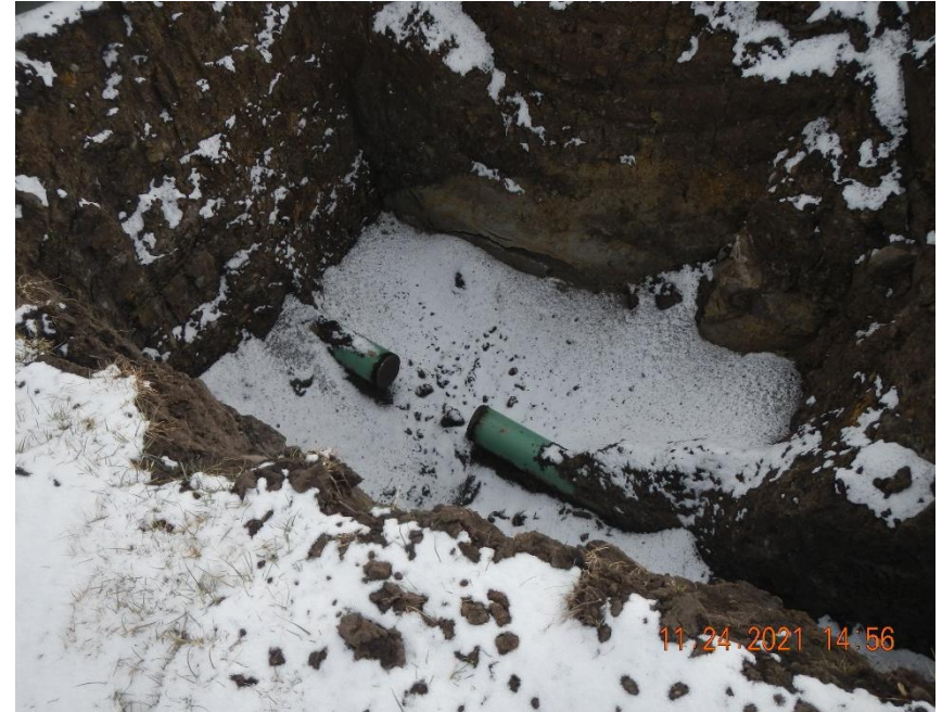
Flow line with caps welded on.
