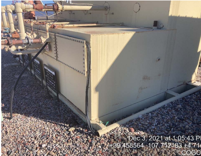
Glycol vessel lacking labeling
