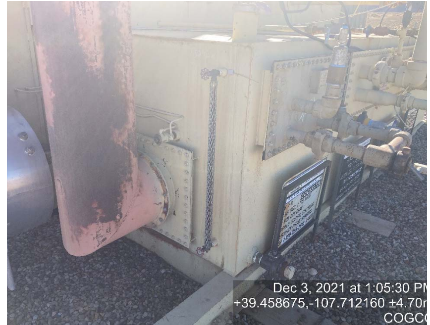
Glycol vessel lacking labeling fluid is seen in sight glass
