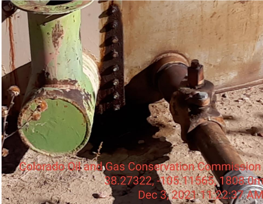
Photo 5 Stained soil under inspection hatch to tank.
