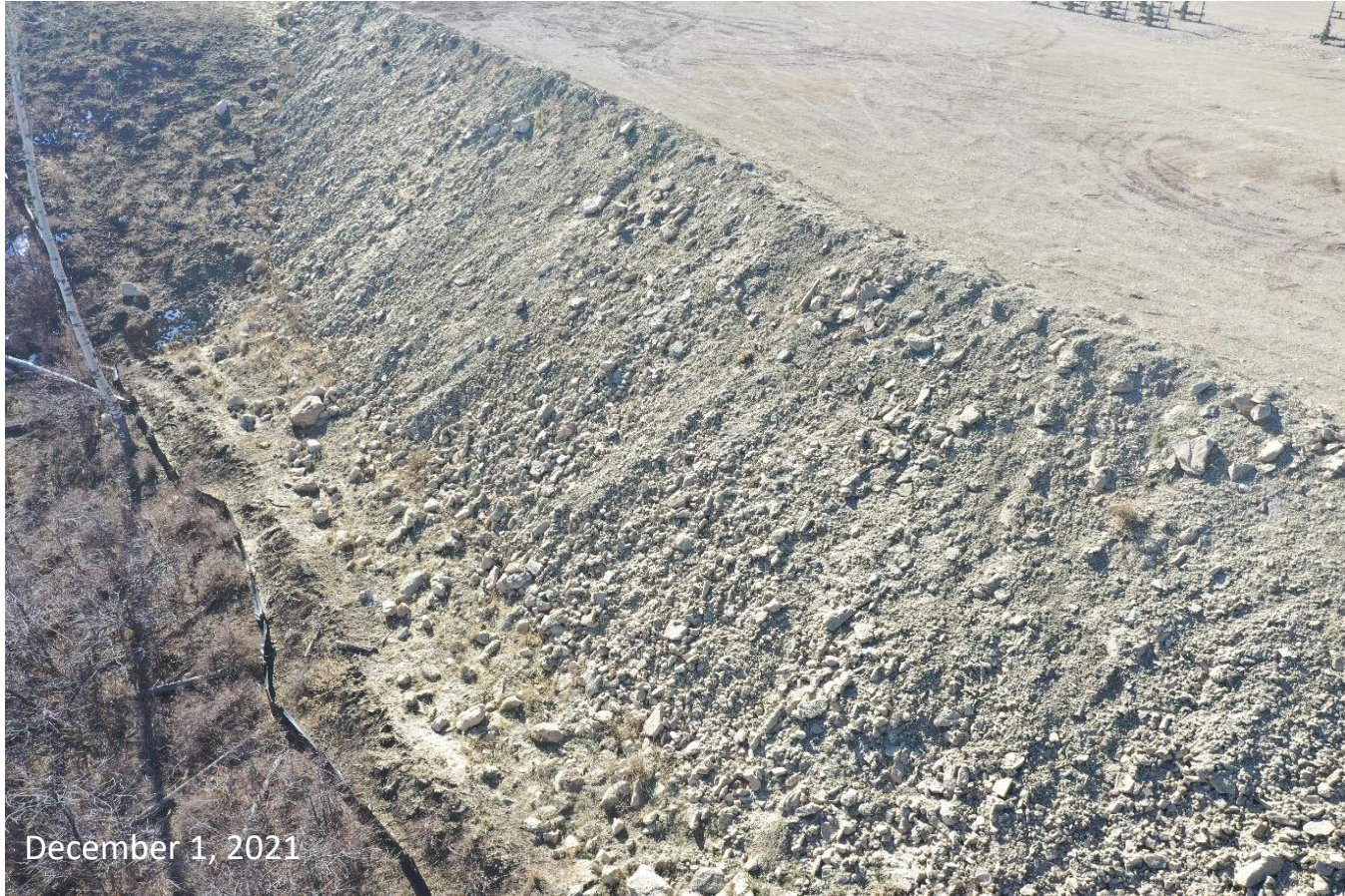
Photo 7: Photo provides example of the fill slopes on the east end of the Location; slopes constructed with a steep grade, with rocky subgrade material. Photo shows control measures to protect/stabilize the slopes of the Location remain missing or insufficient.
