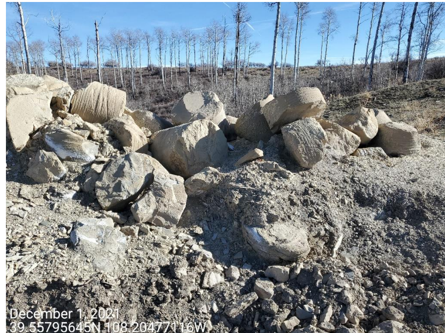
Photo 10: Photos taken from the southeast end of the Location. Photo shows various concrete waste/debris stored and/or partially buried on the southeast end of the Location.
