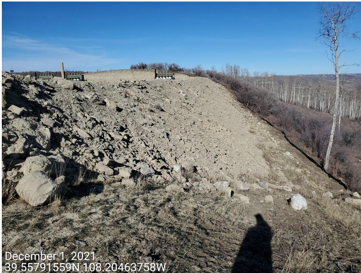
Photo 8: Photo provides example of the fill slopes on the east end of the Location; slopes constructed with a steep grade, with rocky subgrade material. Photo shows control measures to protect/stabilize the slopes of the Location remain missing or insufficient.
