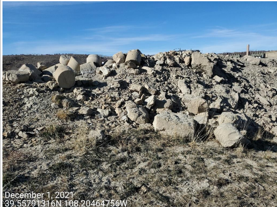
Photo 9: Photos taken from the southeast end of the Location. Photo shows various concrete waste/debris stored and/or partially buried on the southeast end of the Location.
