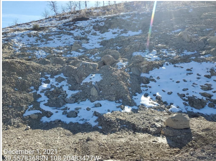
Photo 11: Photos taken from the southeast end of the Location. Photo shows various concrete waste/debris stored and/or partially buried on the cut slope.
