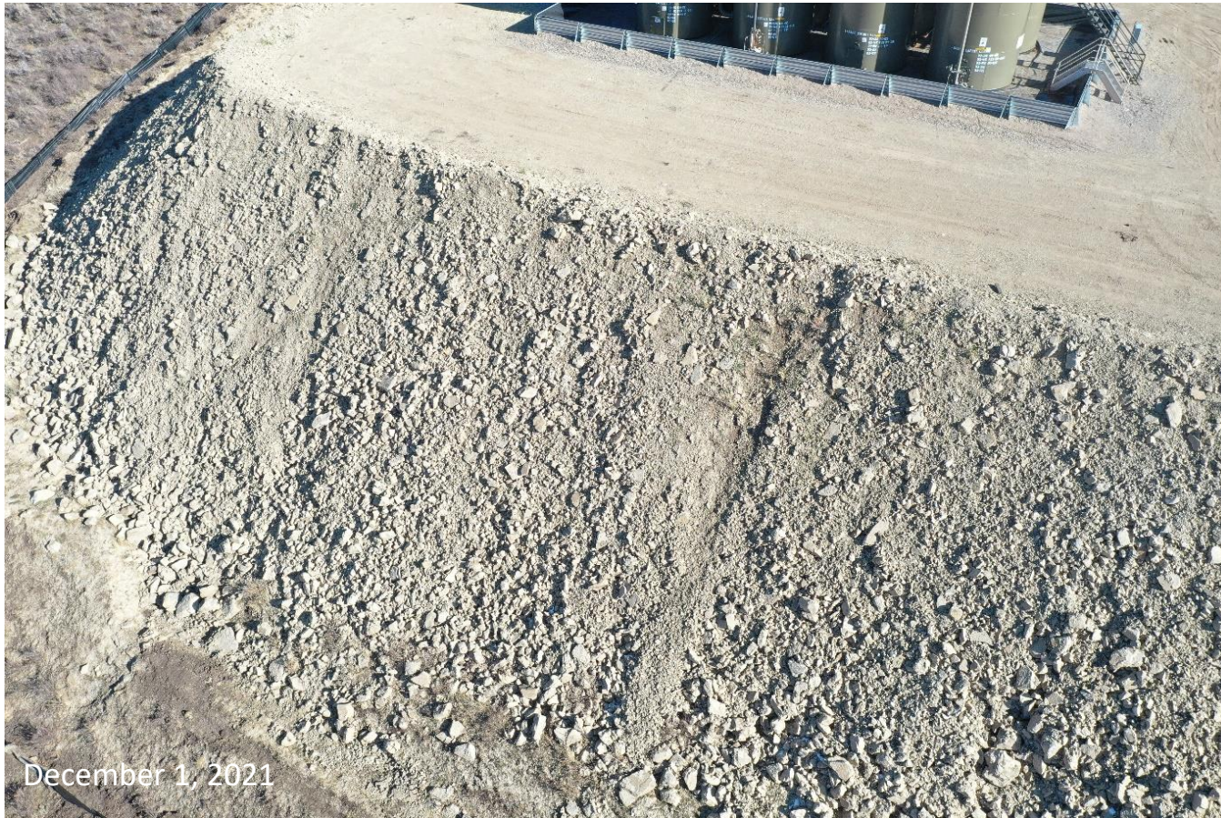
Photo 5: Photo provides example of the fill slopes on the west end of the Location; slopes constructed with a steep grade, with rocky subgrade material. Photo shows control measures to protect/stabilize the slopes of the Location remain missing or insufficient.
