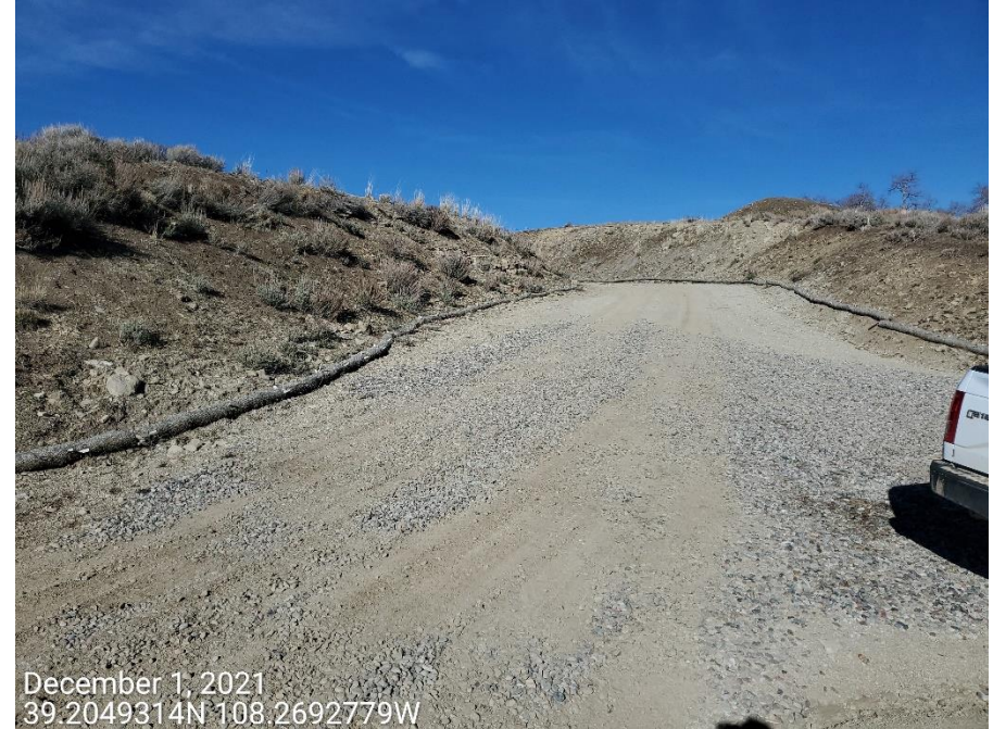
Photo 8: Photos taken from the two access road entrances on the southeast end of the Location. Photos examples showing control measures to stabilize the Location, and minimize tracking and offsite sediment transport are inadequate, and have not been installed/maintained in proper functioning condition per good engineering practices; tracking and sediment transport observed. Photo left also shows second access road has not been reclaimed.
