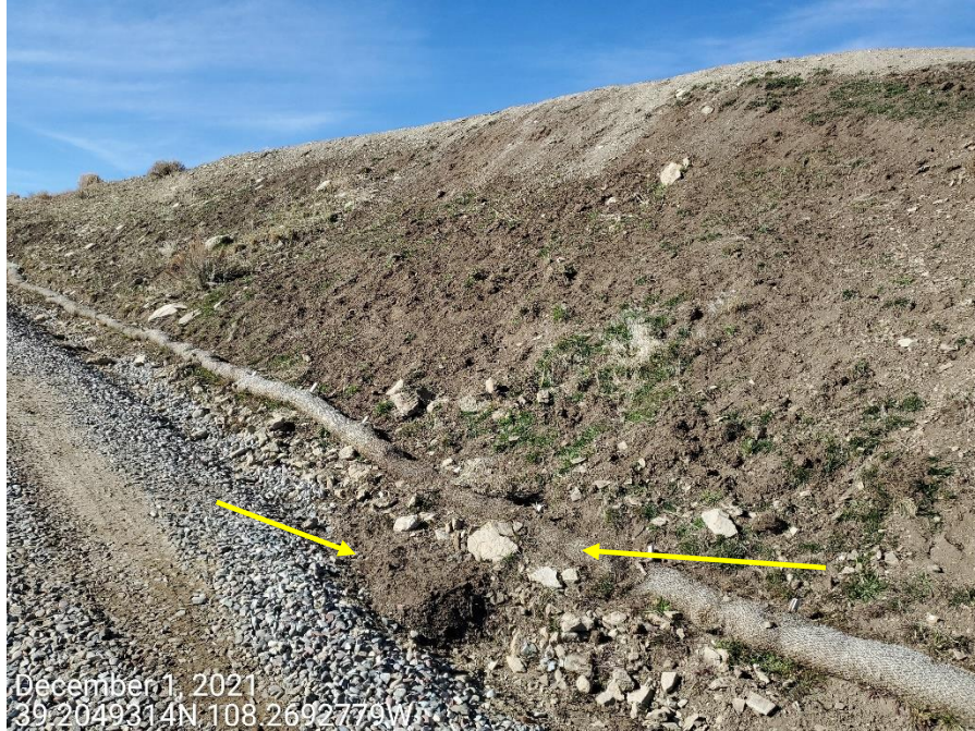
Photo 6: Photo taken from the slopes on the southeast end of the Location. Though rill erosion previously observed appears to have been repaired, control measures to protect and stabilize the slopes remaining missing or insufficient. Arrow shows sediment discharge due to un-stabilized slopes.
