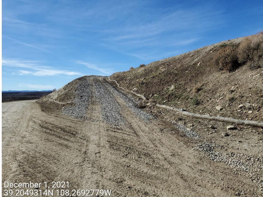
Photo 8: Photos taken from the two access road entrances on the southeast end of the Location. Photos examples showing control measures to stabilize the Location, and minimize tracking and offsite sediment transport are inadequate, and have not been installed/maintained in proper functioning condition per good engineering practices; tracking and sediment transport observed. Photo left also shows second access road has not been reclaimed.
