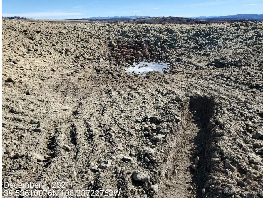
Photo 4: Sediment trap has been re-constructed with an appropriate engineered outlet.
