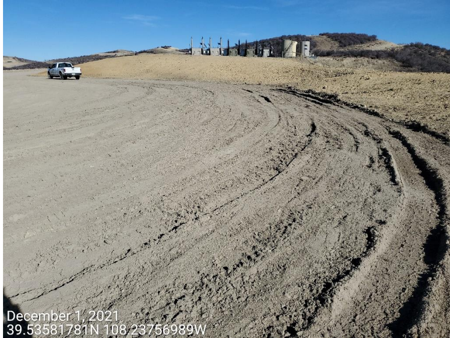
Photo 3: Photo taken from the east end of the Location. Photo provides example showing control measures to stabilize the entire Location, minimize tracking and offsite sediment transport per good engineering practices remain missing or insufficient.
