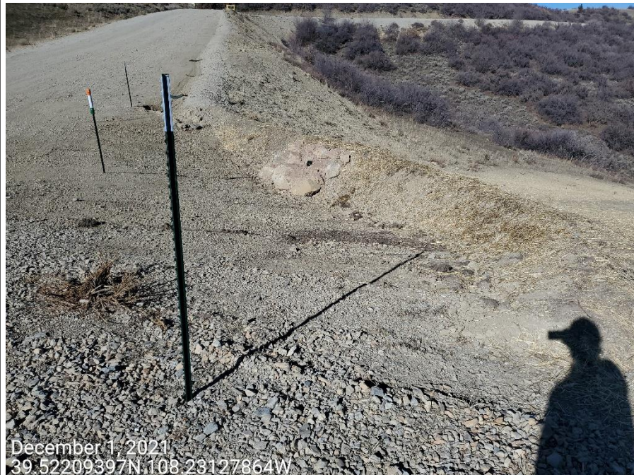
Photo 1: Photos taken from the northwestern end of the Location, facing west and north. Photos show Operator has installed a sediment trap in conjunction with a slope drain; erosion degradation repaired.
