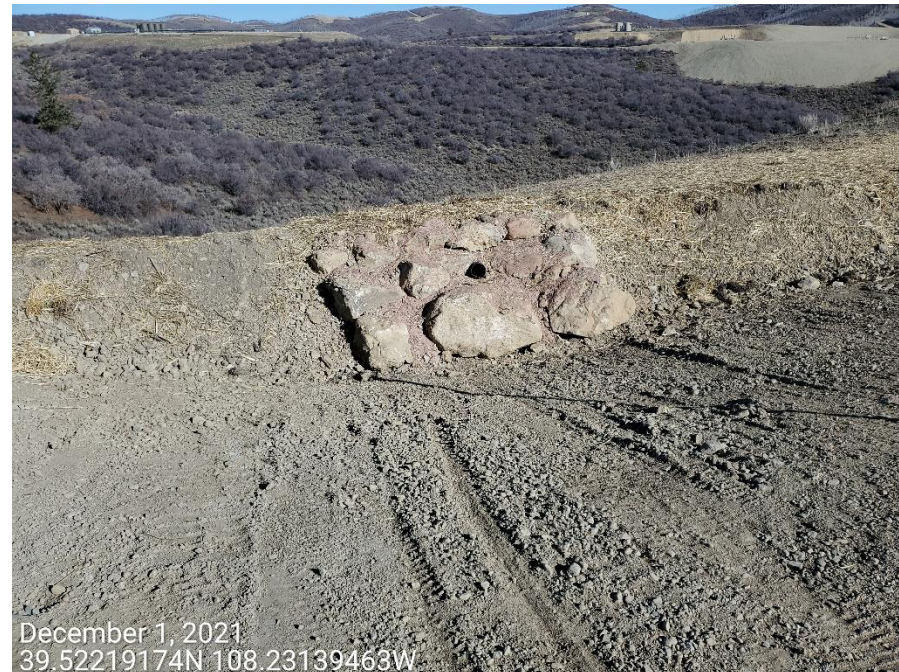
Photo 1: Photos taken from the northwestern end of the Location, facing west and north. Photos show Operator has installed a sediment trap in conjunction with a slope drain; erosion degradation repaired.
