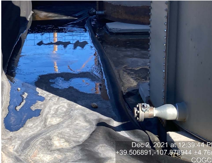
Load lines missing bull plugs/caps
