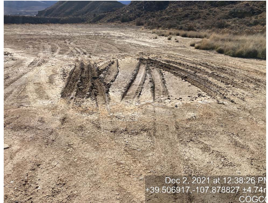
lack of stabilization/compaction
