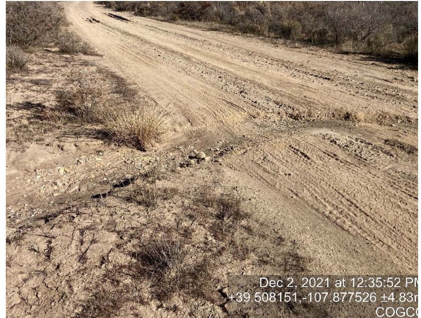
Access road lack of stabilization/compaction
