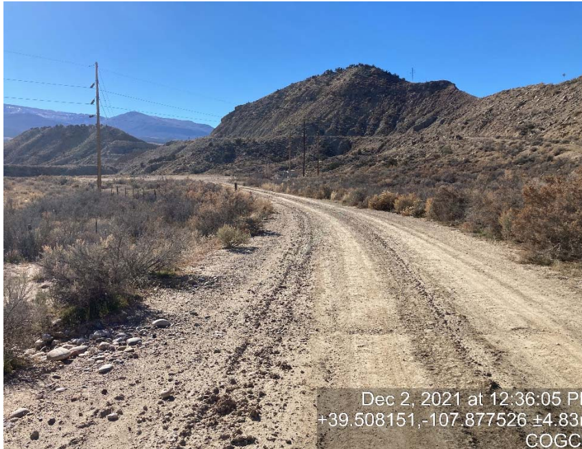
Access road lack of stabilization/compaction
