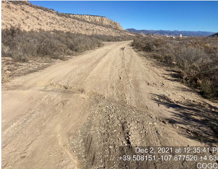
Access road lack of stabilization/compaction
