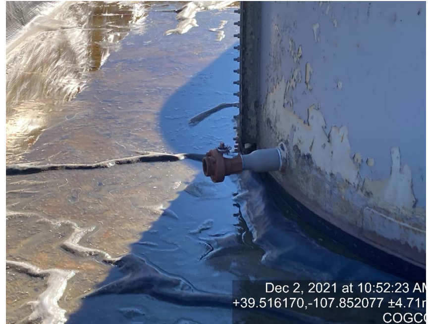
Load line missing bull plug/cap
