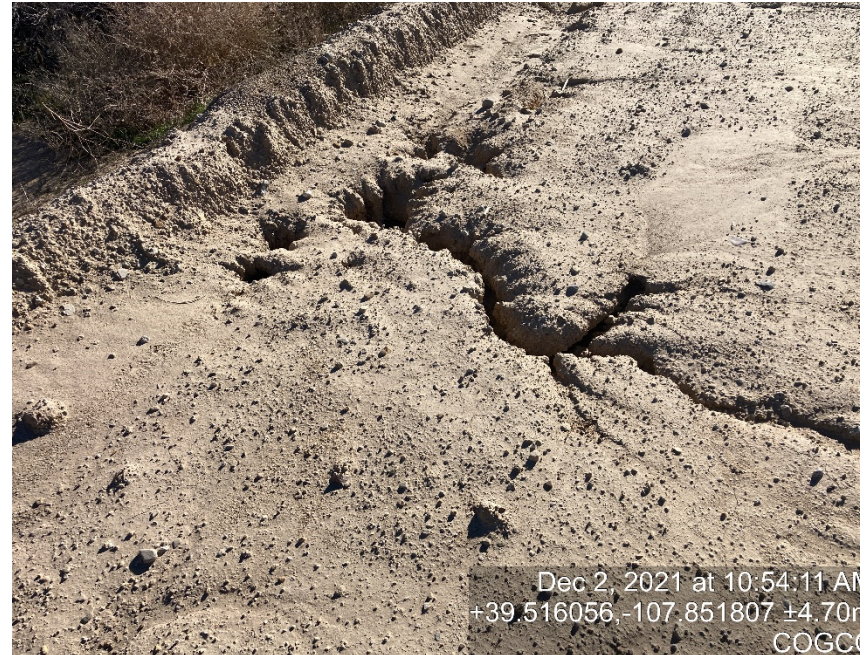
Erosion leading to the tunneling under berm.
