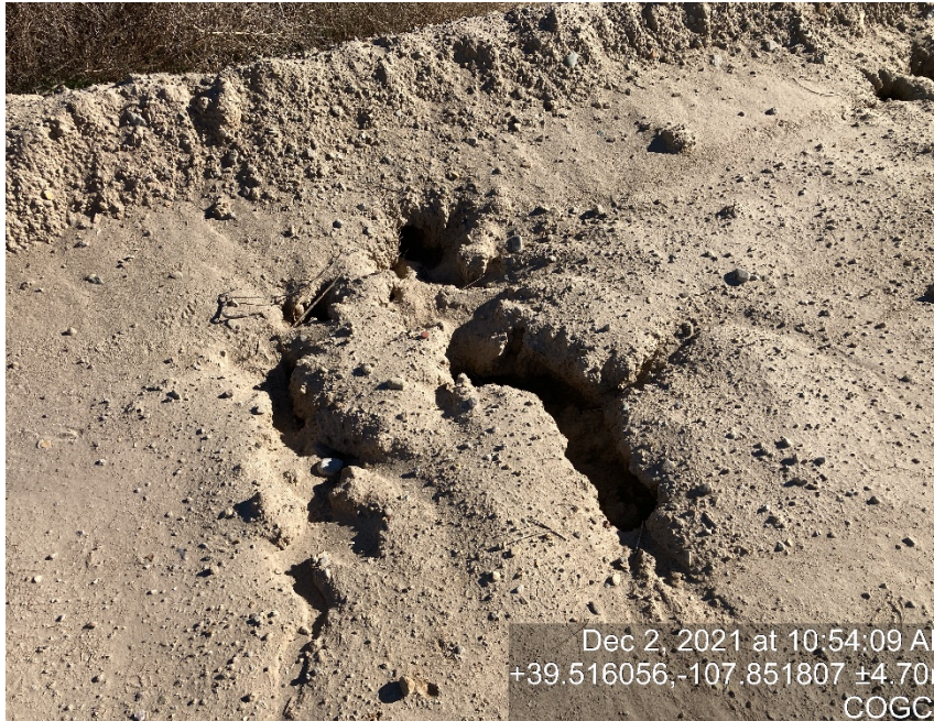
Erosion leading to the tunneling under berm.
