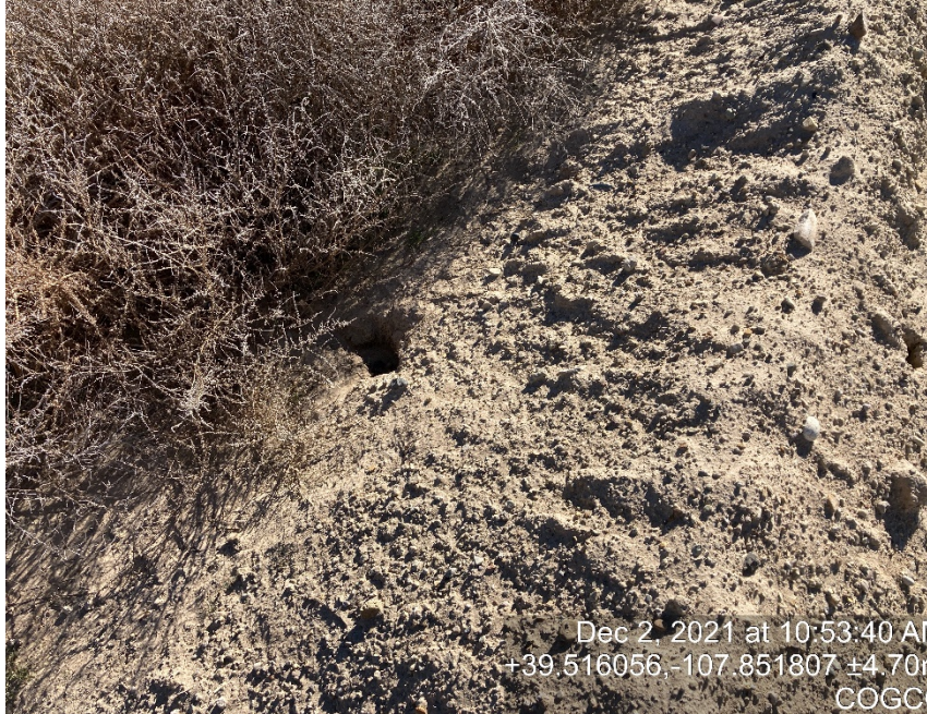
One spot of the outlet side of tunneling through berm
