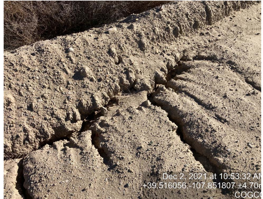
Erosion leading to the tunneling under berm.
