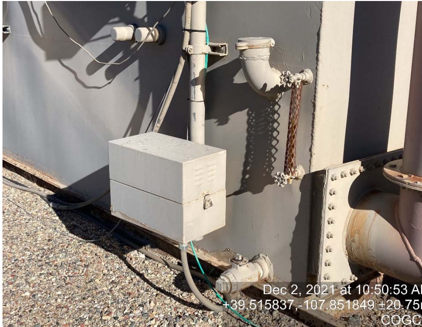
Glycol vessel lacking labeling
