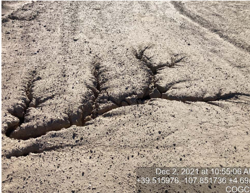
Erosion leading to the tunneling under berm.
