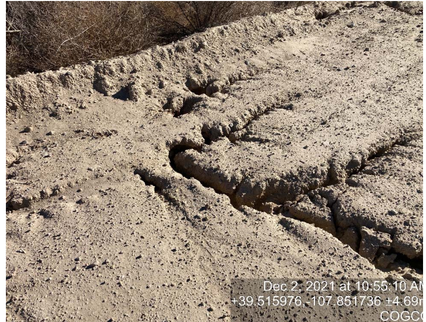
Erosion leading to the tunneling under berm.
