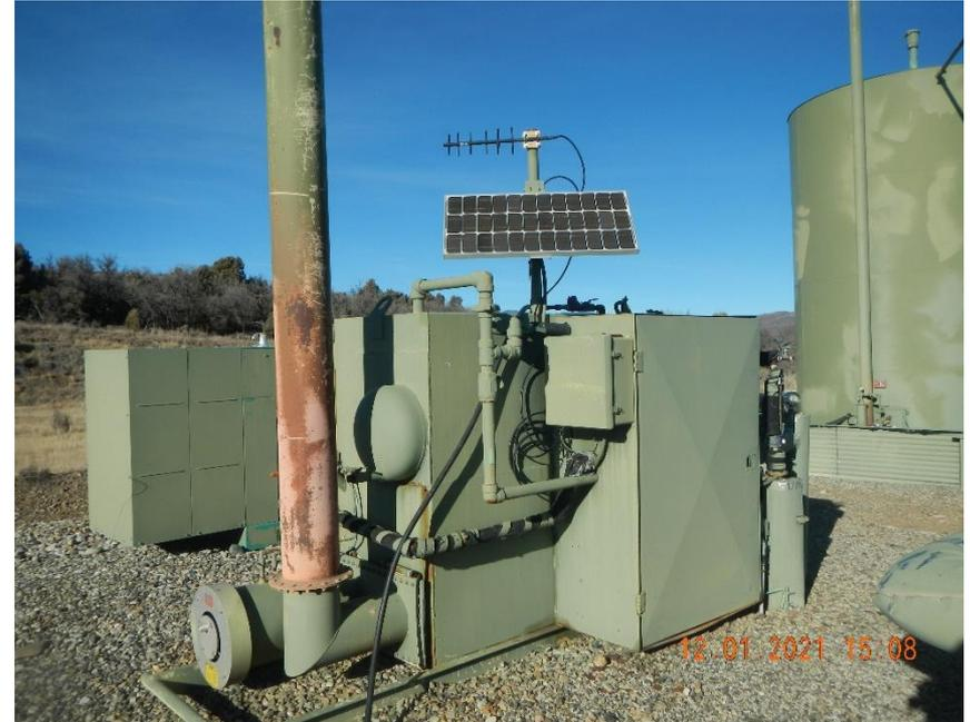
**Heated separator has a glycol storage tank with no labeling.**
