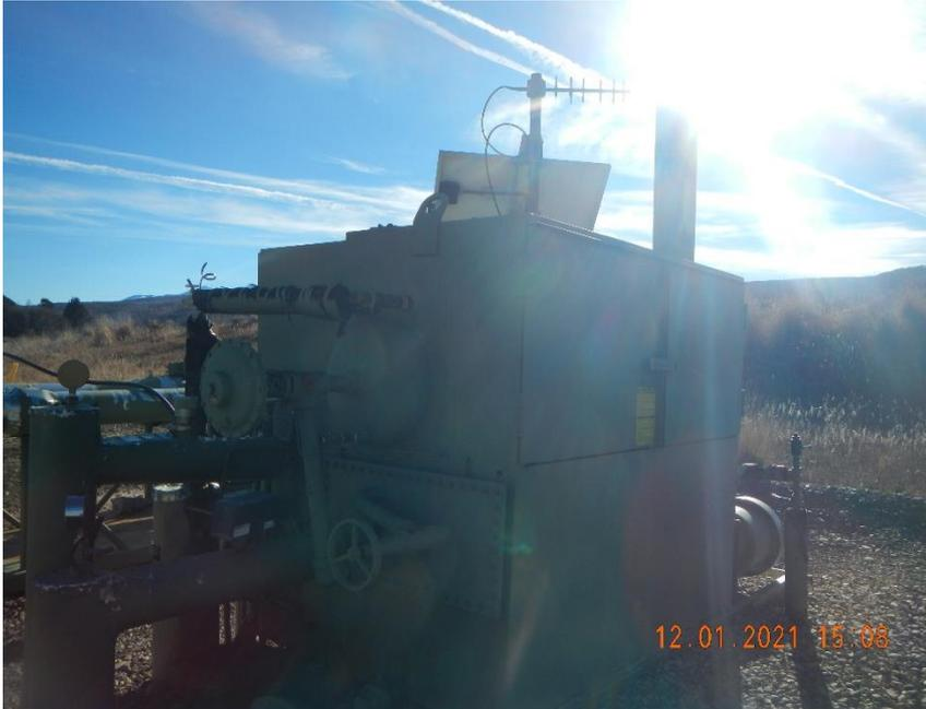
**Heated separator has a glycol storage tank with no labeling.**
