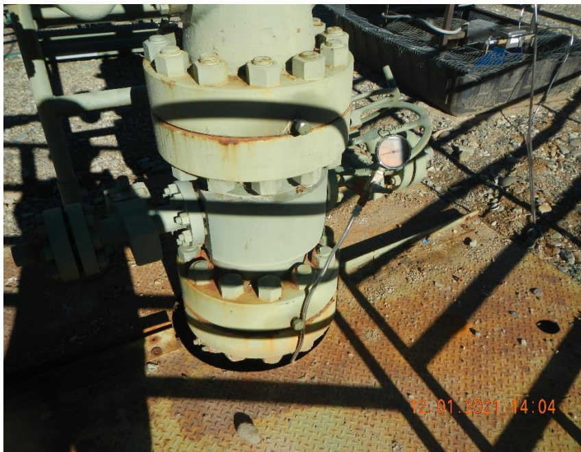
Braden access and gauge plumbed to above ground surface.
