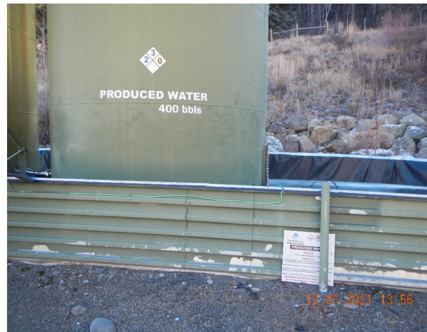
NFPA label colors are faded on tanks.
