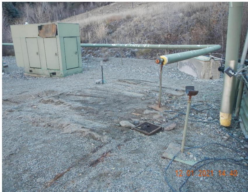
Square metal catch container in front of removed pump house has not been removed.
