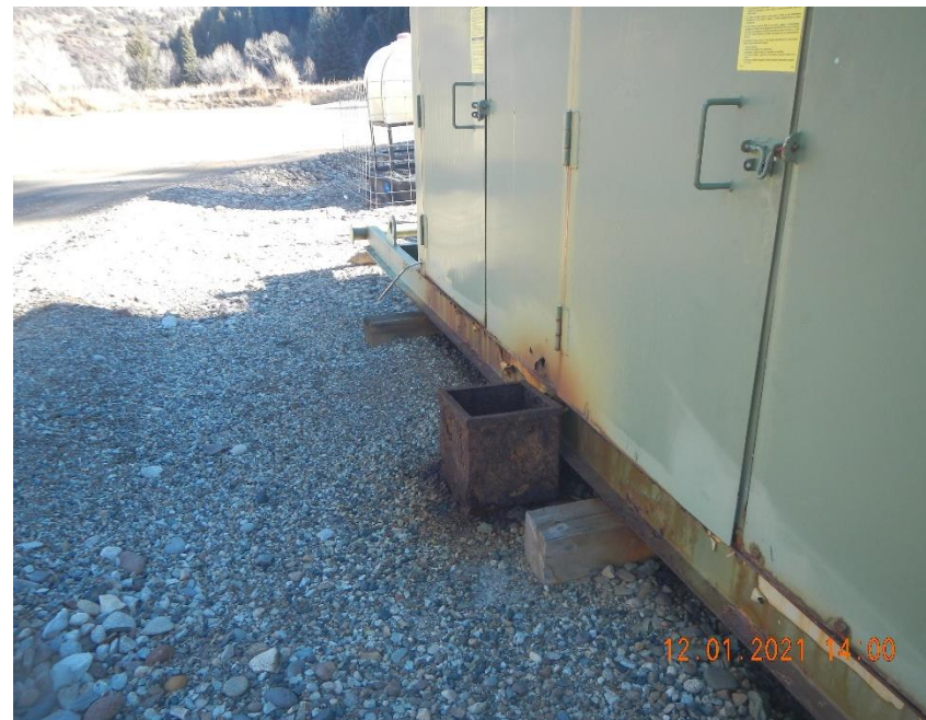
Square metal catch container in front of separator is rusted and deteriorating.
