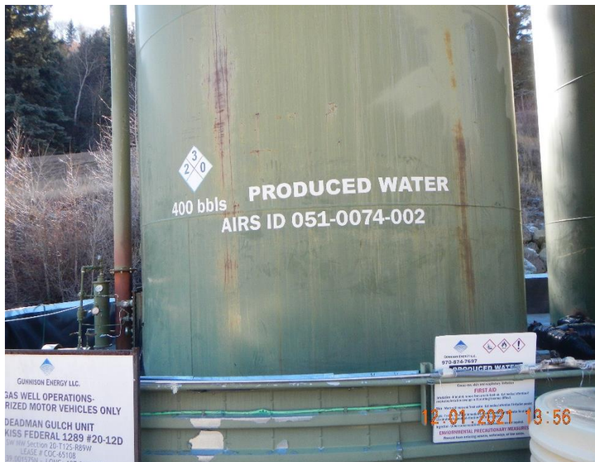
NFPA label colors are faded on tanks.
