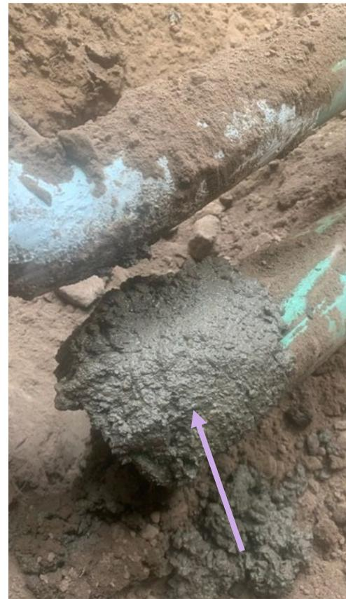
The abandonment work for the indicated flowline was completed on 11/16/2021 and 11/23/2021 with capping of both line ends including a cement plug. See photo documentation.
