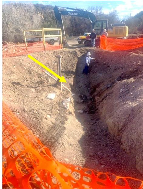
The abandonment work for the indicated flowline was completed on 11/18/2021 and 11/23/2021 with capping of both line ends including a cement plug. See photo documentation.
