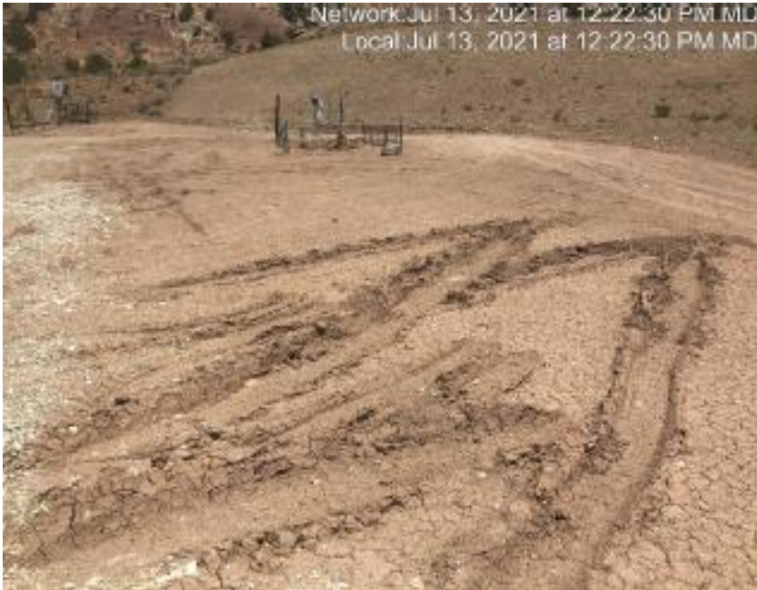
Photo #4407 from inspection #699803393 conducted on 7/13/21.
