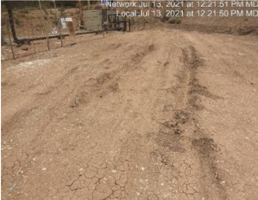
Photo #4406 from inspection #699803393 conducted on 7/13/21.
