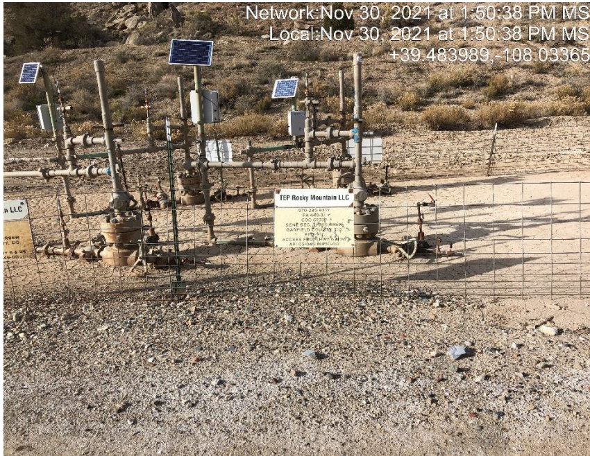
Photo #5293 Wellhead sign weathered and not legible.
