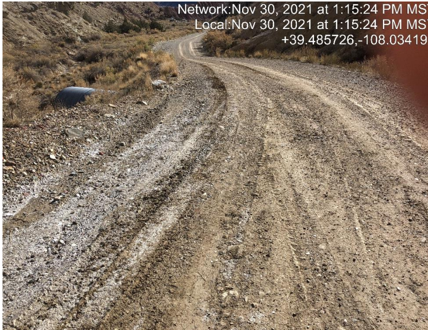
Photo #5291 Insufficient tracking BMP at entrance to location.
