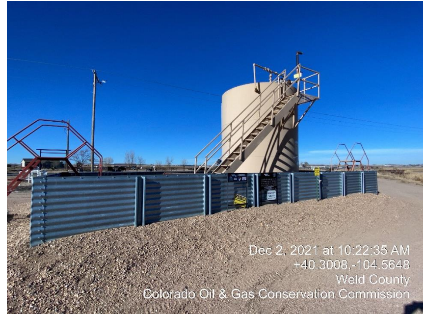
Photo #2 Tank Battery
