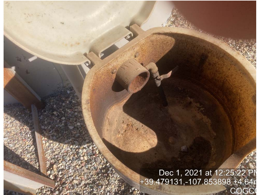
Load lines missing bull plugs/caps
