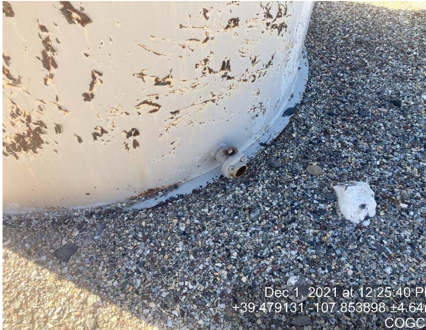
Load lines missing bull plugs/caps
