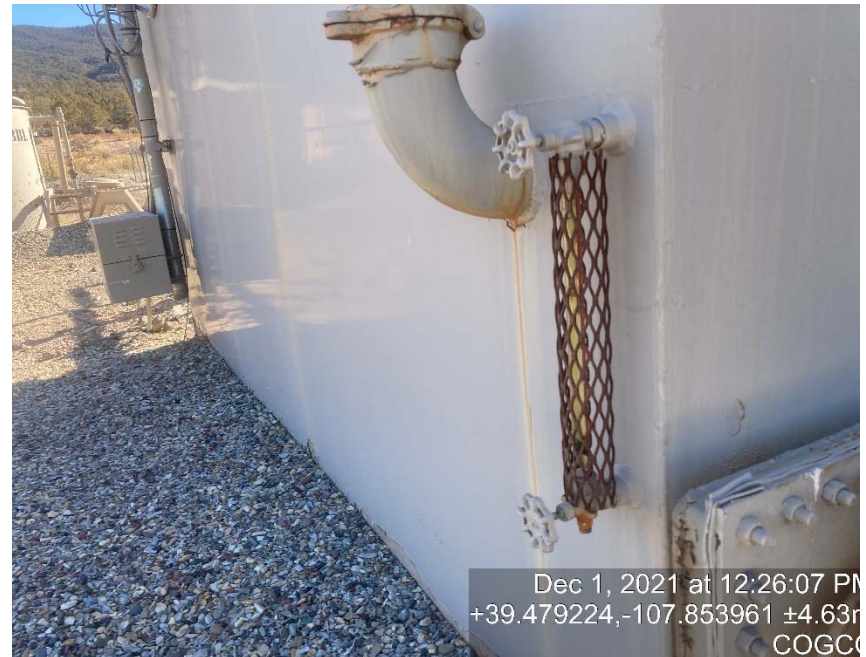
Glycol vessel not properly labeled, as seen in sight glass the fluid.
