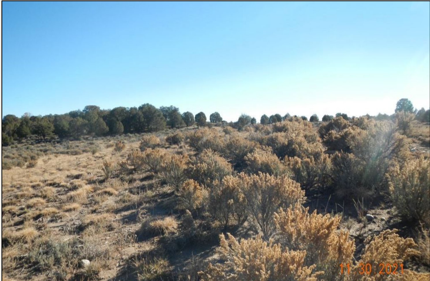
Photo 2. View of the northern fill slope from the northwestern corner facing eastward. Revegetation is progressing with big sagebrush, western wheatgrass, Indian ricegrass, and sand dropseed.
