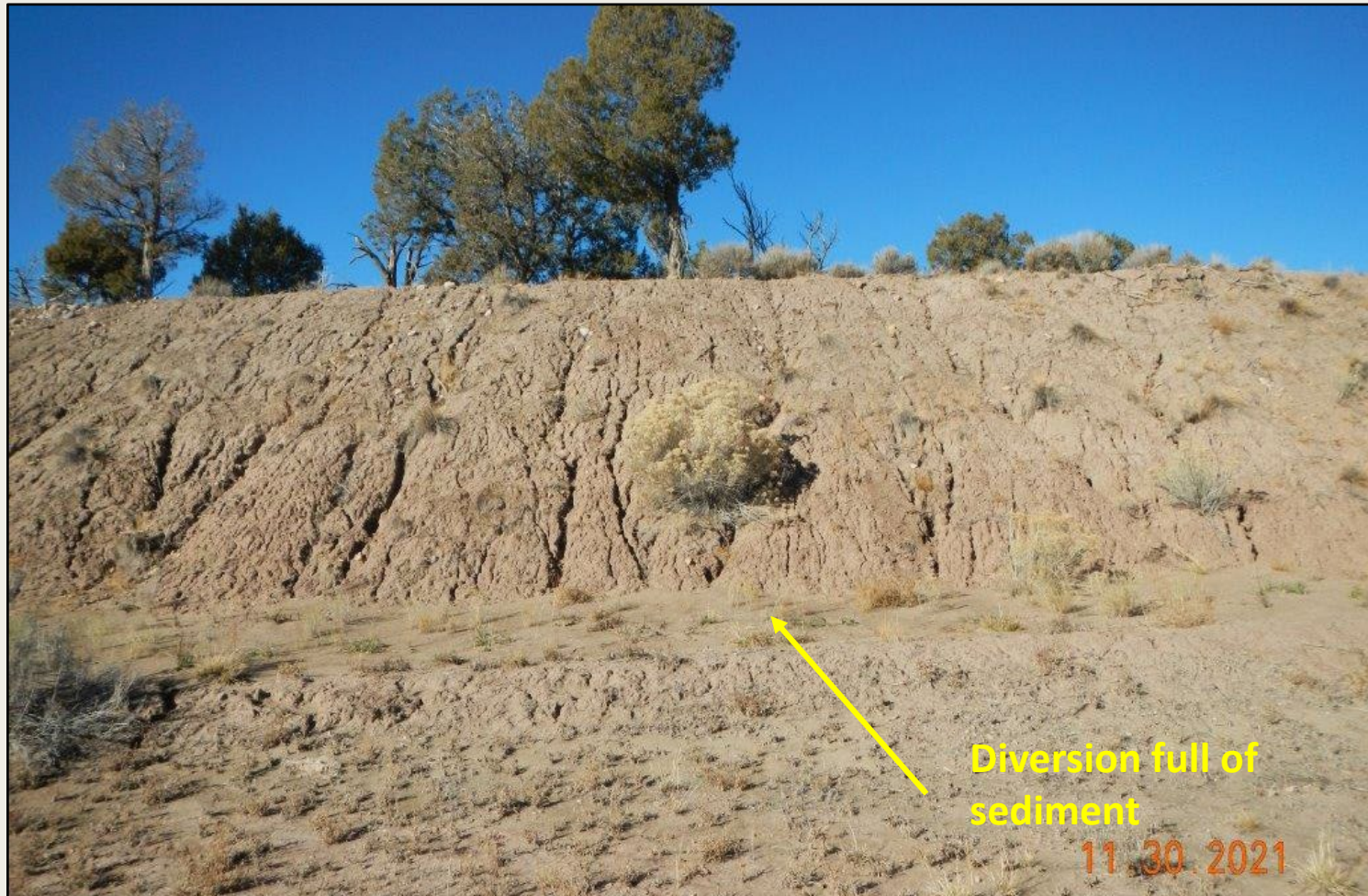
Photo 3. View of the western cut-slope. Slope is not stabilized, with rills approximately 8-12 inches deep. Diversion ditch is full of sediment.
