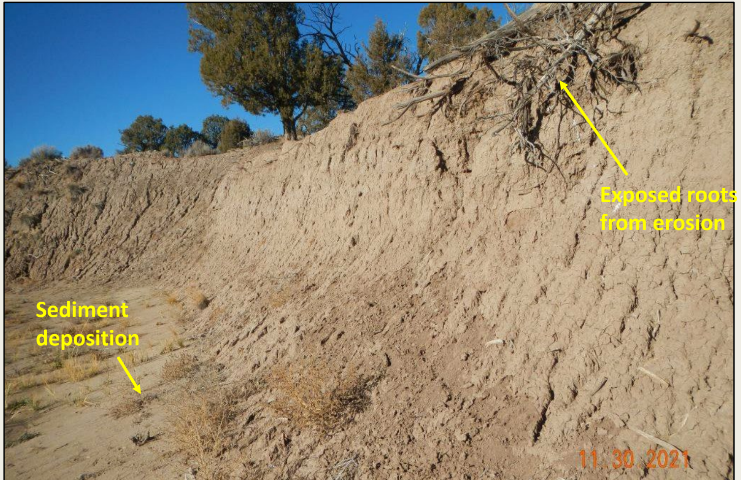
Photo 4. View of the northern cut-slope. Bare soils on steep slope need stabilization.
