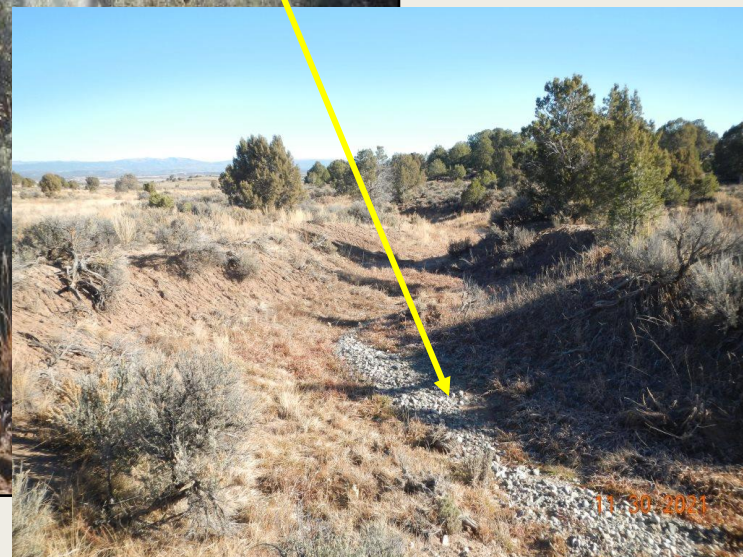
Photo 6. View of area approx. 50 ft down-slope of culvert outlet, where significant volumes (approx. 75ft long, 4-6 ft wide, and 4-6 inches deep) observed within the streambed.
