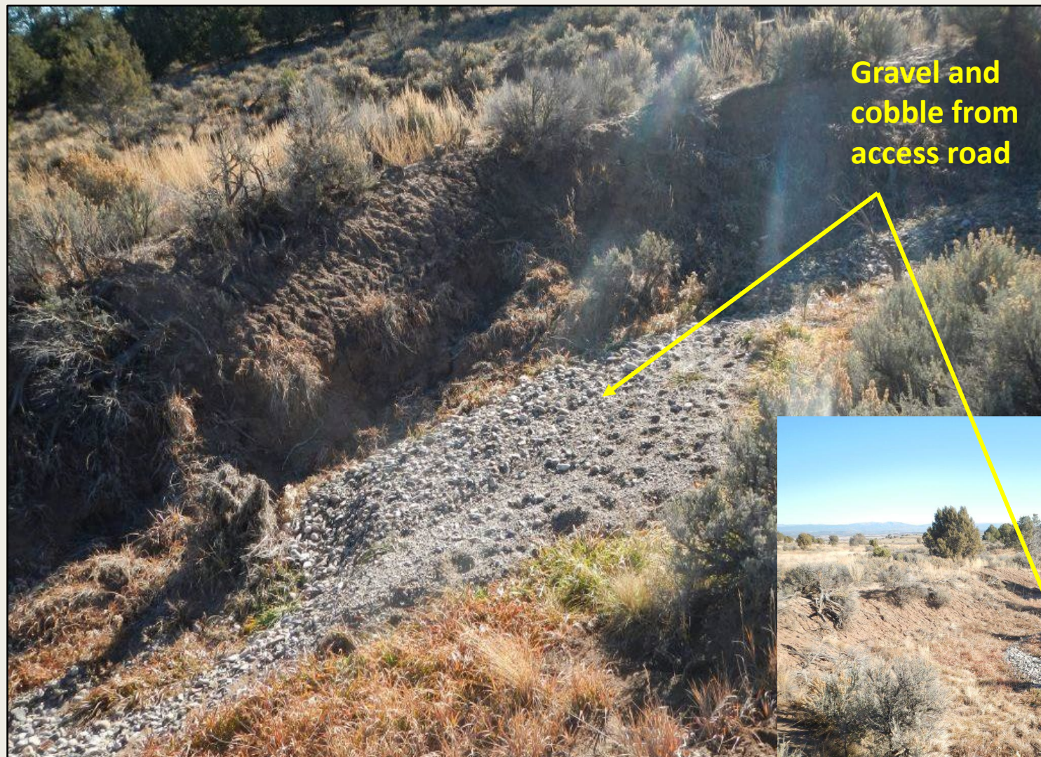
Photo 6. View of area approx. 50 ft down-slope of culvert outlet, where significant volumes (approx. 75ft long, 4-6 ft wide, and 4-6 inches deep) observed within the streambed.
