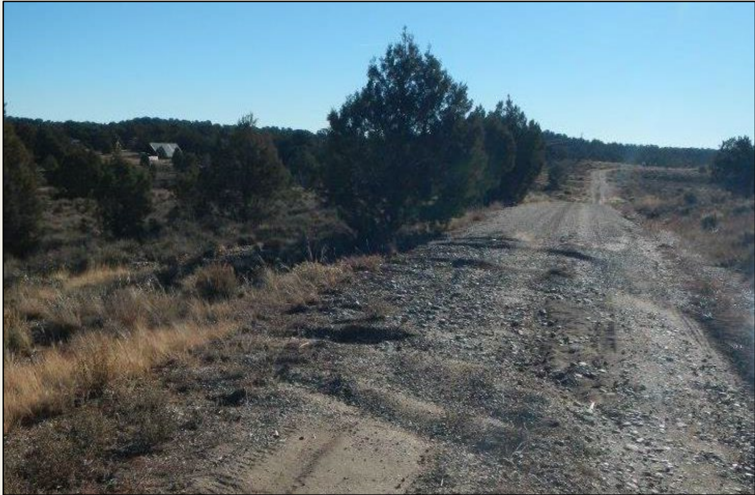
Photo 3. View of erosional scouring and erosion on the access road where stormwater flows are improperly diverted. Approximately 4-6 inches deep of material is eroded off of the road and down-slope.
