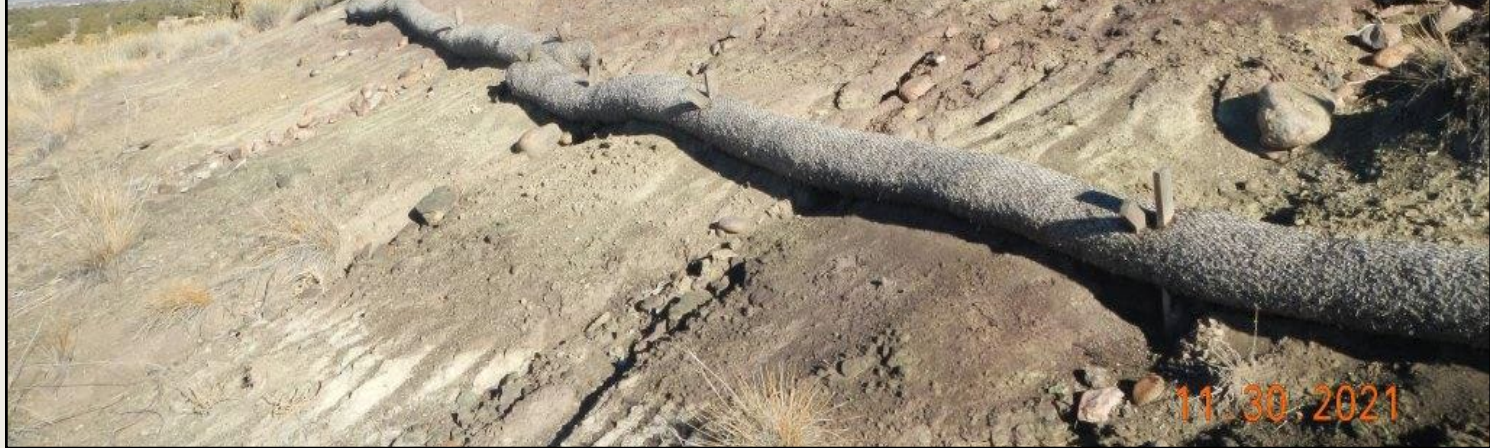
Photo 4. View of bare/unstabilized soils on the eastern cut-slope. Wattles are not adequate BMPs here.
