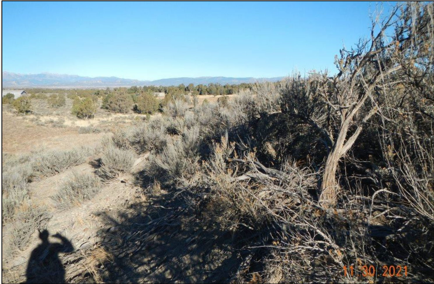
Photo 2. View of the western fill slope, from the southwestern corner facing northward. Revegetation is progressing with sagebrush, western wheatgrass, and Indian ricegrass.
