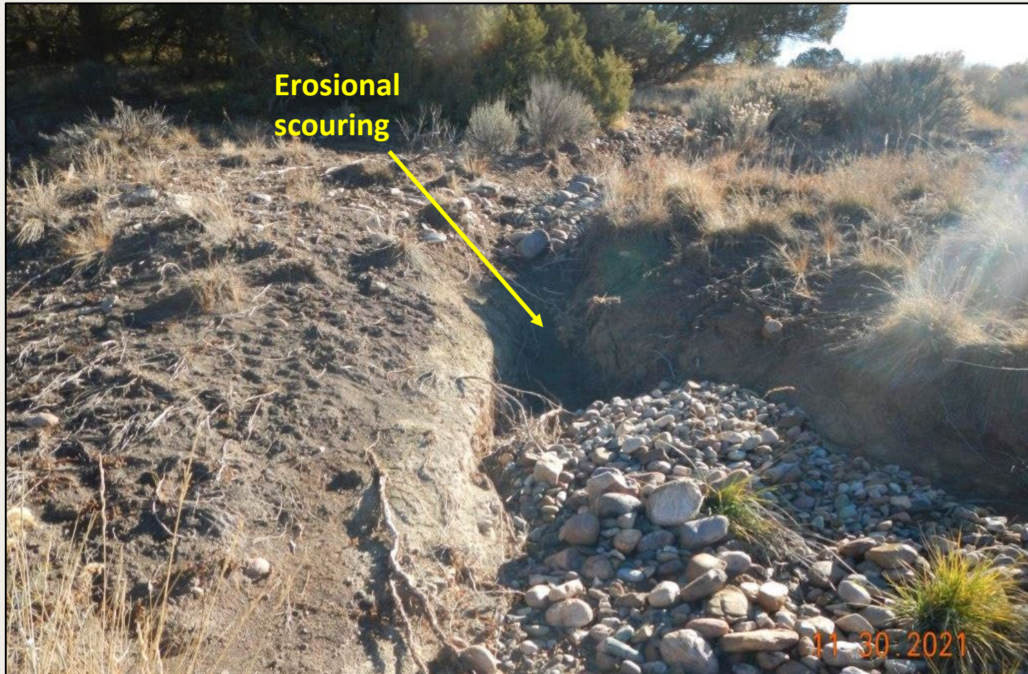
Photo 3. View of erosional scouring within diversion channel in southeastern project area. Cobble and sediment are washed down-slope from the diversion.
