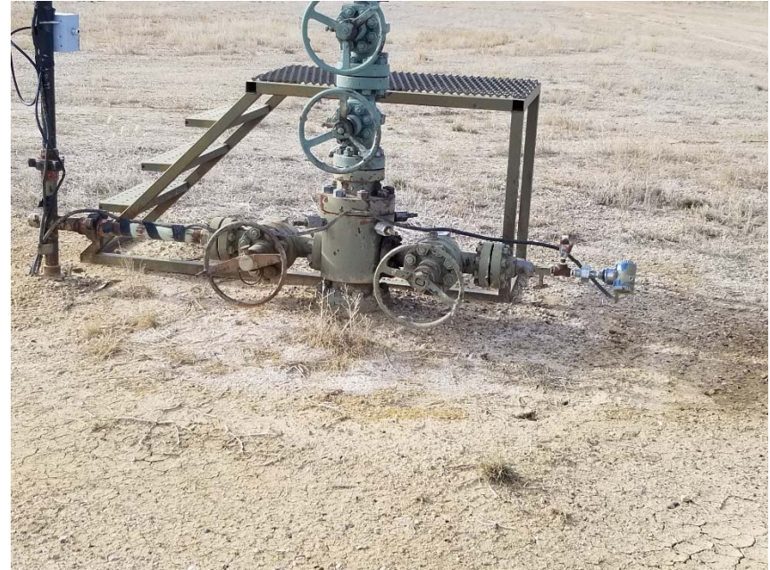
Photo 2. No bradenhead access apparent.
