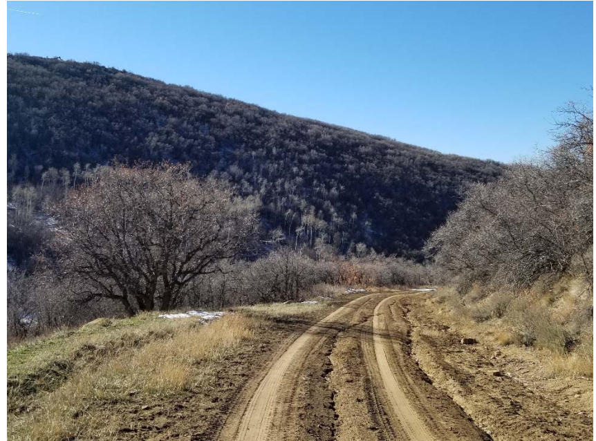
Photo 2. Example of sediment migration on access road.
