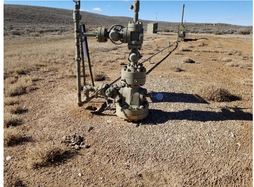
Photo 2. No bradenhead access apparent.
