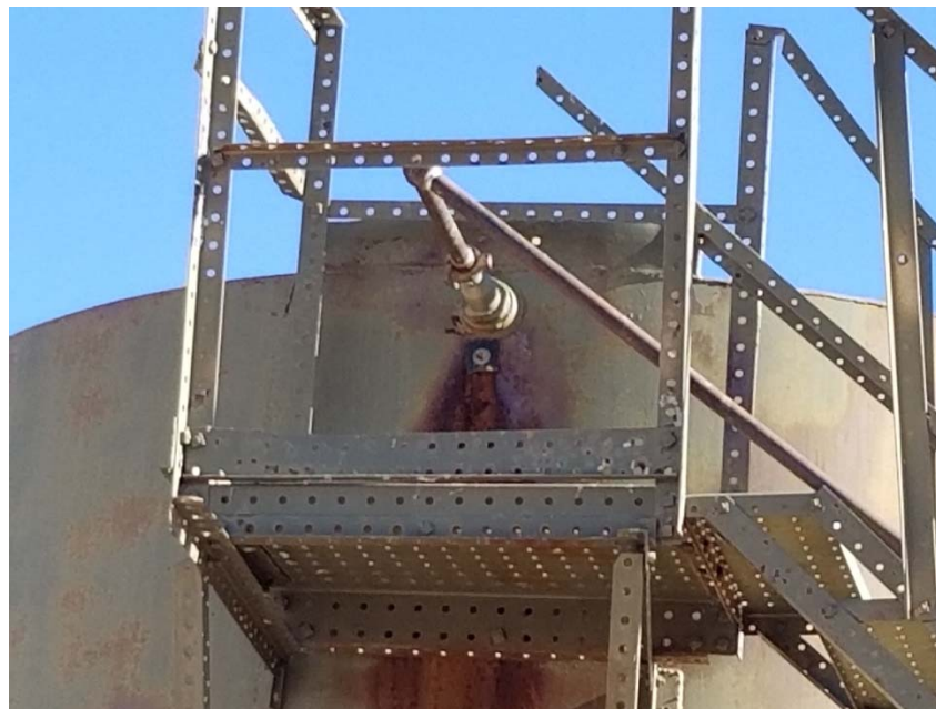
Photo 4. Holes in tank.
