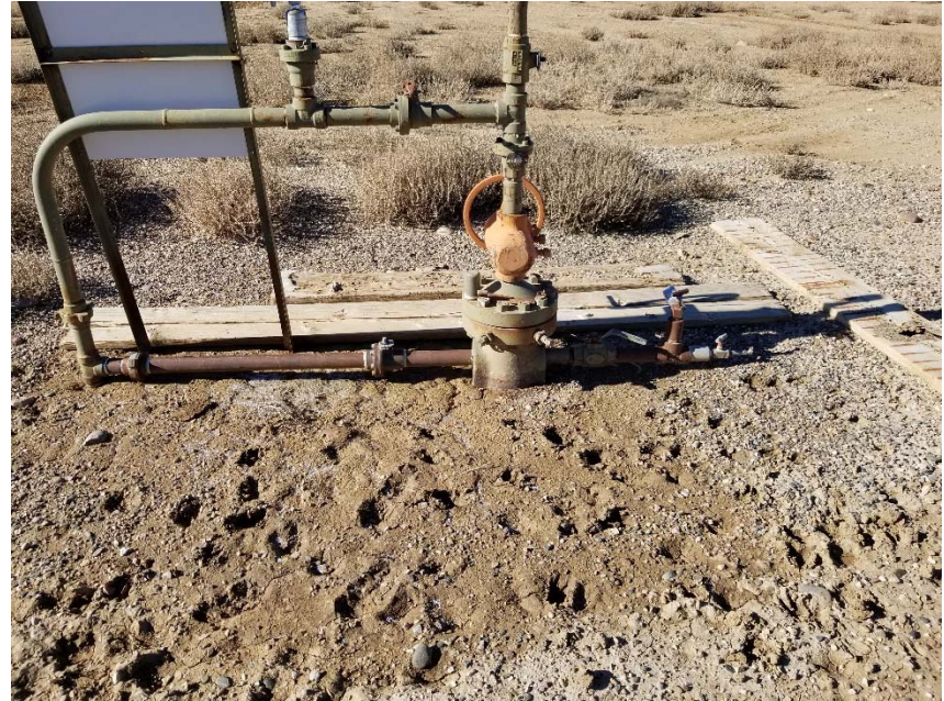
Photo 2. No bradenhead access apparent.
