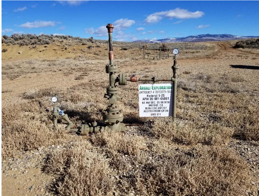
Photo 3. No bradenhead access apparent. Dried annual weeds.
