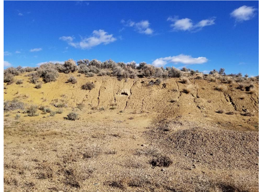
Photo 4. Sediment migration onto location. No stormwater BMPs apparent.
