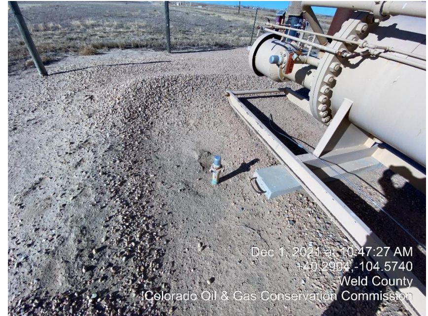
Photo #3 Unmarked Riser
