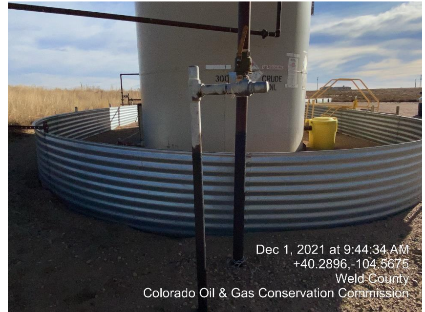
Photo #3 Unmarked Riser
