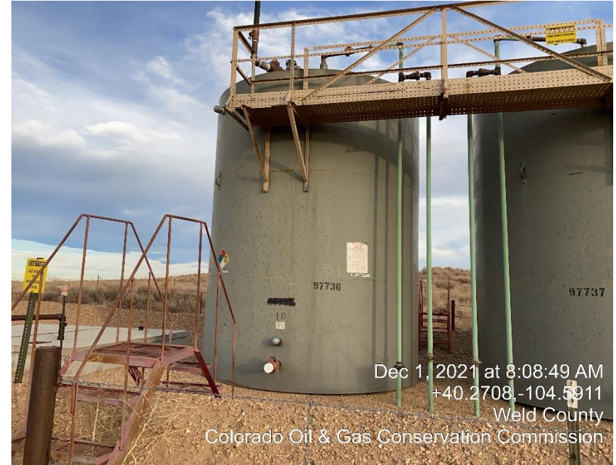
Photo #2 West production tank is missing capacity label and needs replaced
