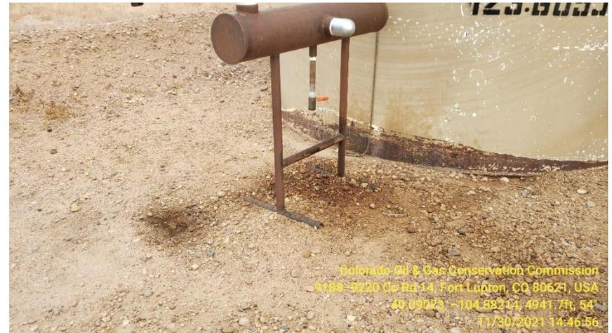
**Photo 7 Stained soil under TB load line**
