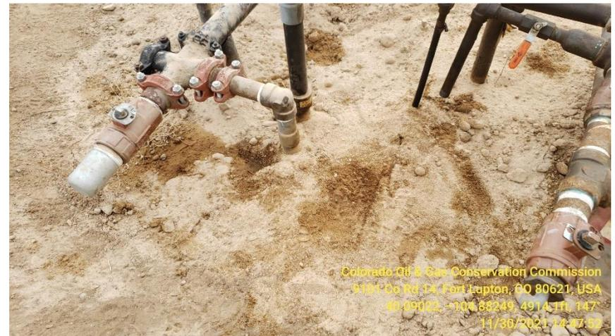
**Photo 9 flow line manifold and aux. pump**
