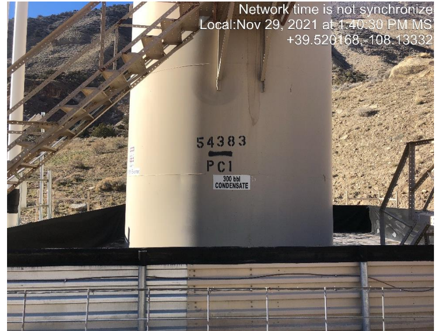
Photo #5279 Condensate tank missing required information.
