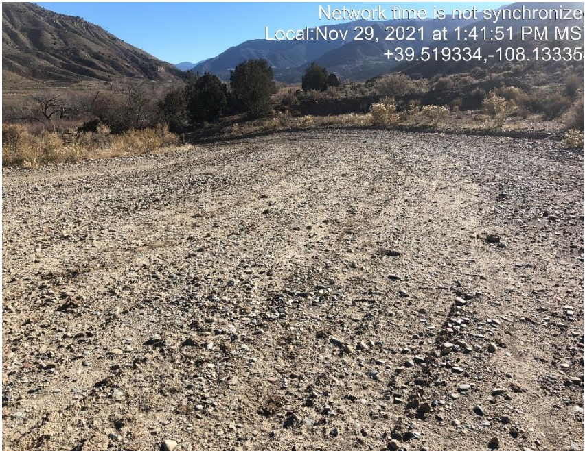
Photo #5280 No form of tracking BMP at entrance to location.
