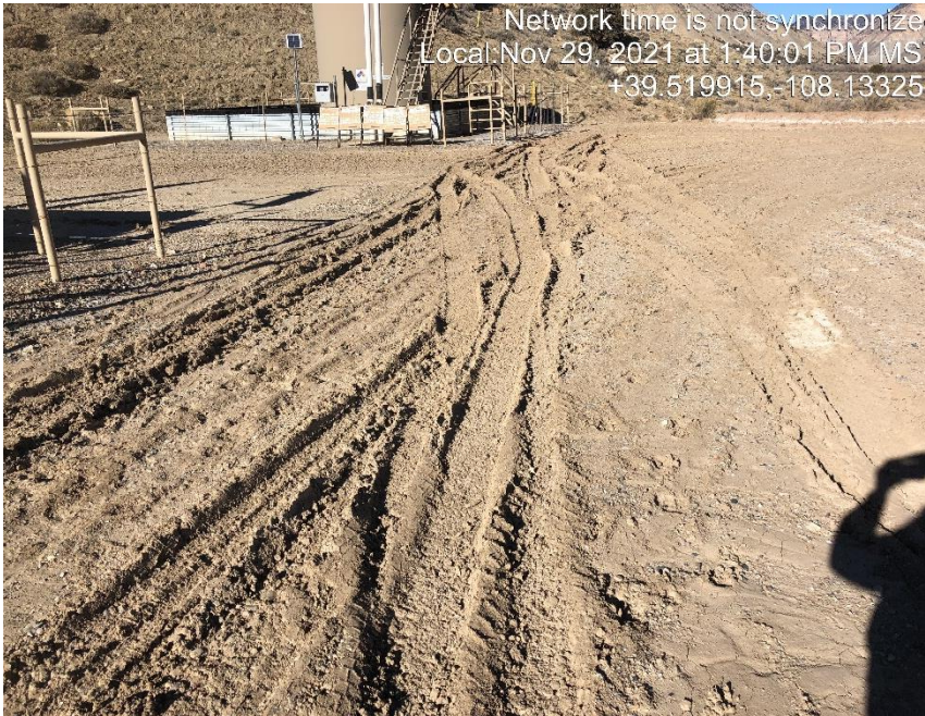
Photo #5277 Location lacks stabilization.
