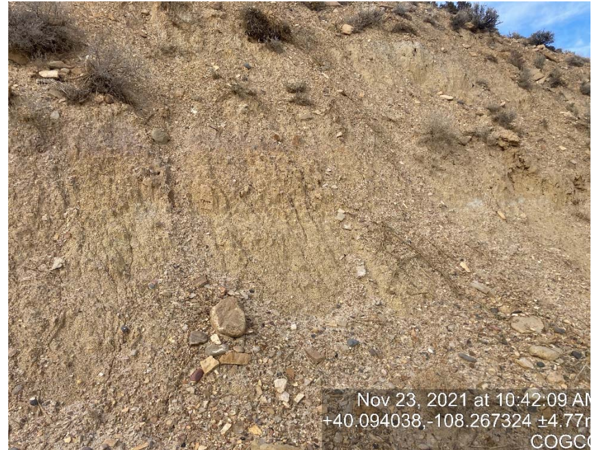
Cut slope not stabilized
