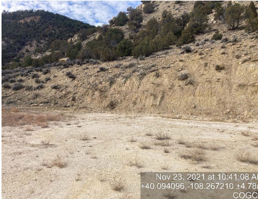
Cut slope not stabilized
