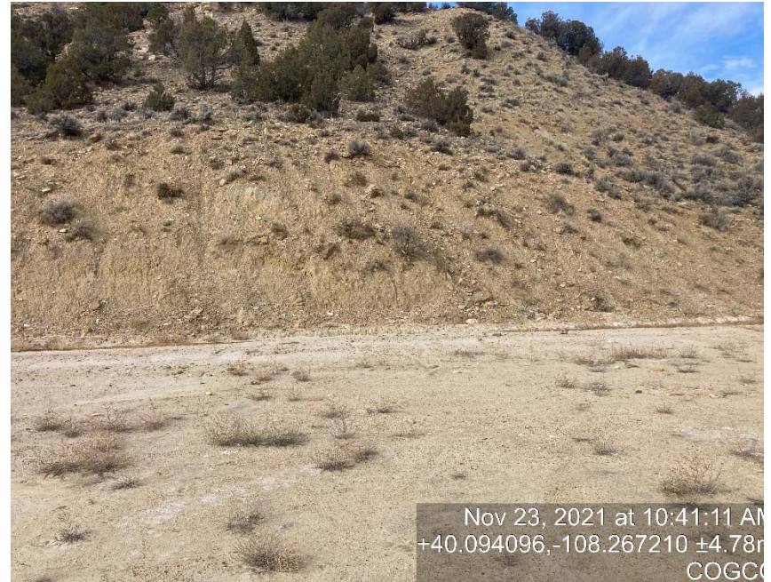
Cut slope not stabilized
