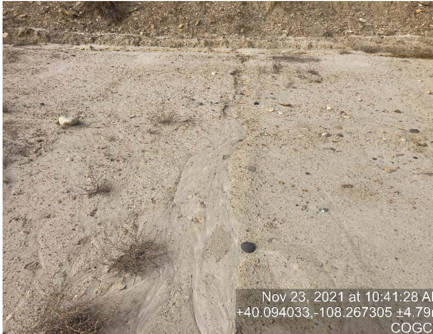
Erosion from cut slope
