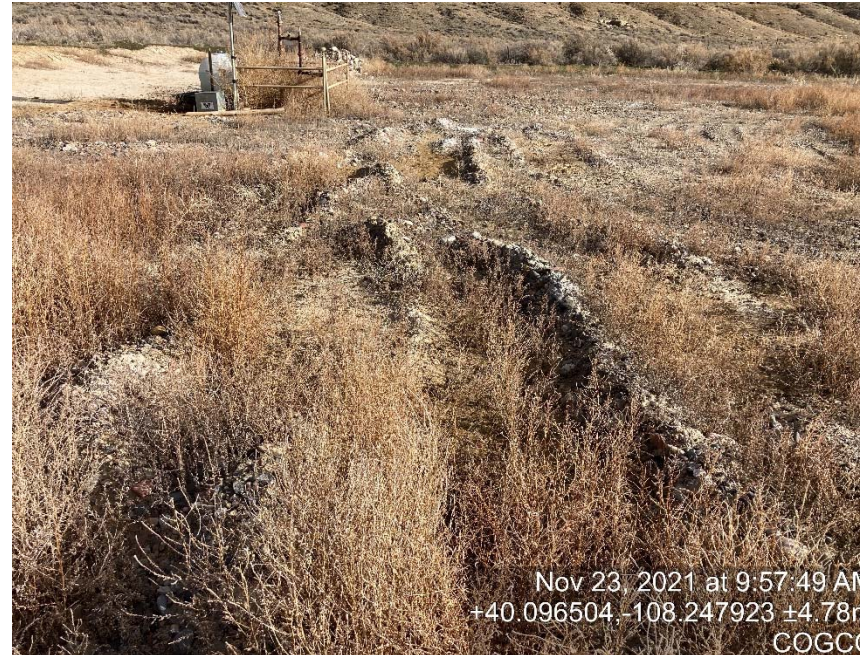
Lack of stabilization/compaction
