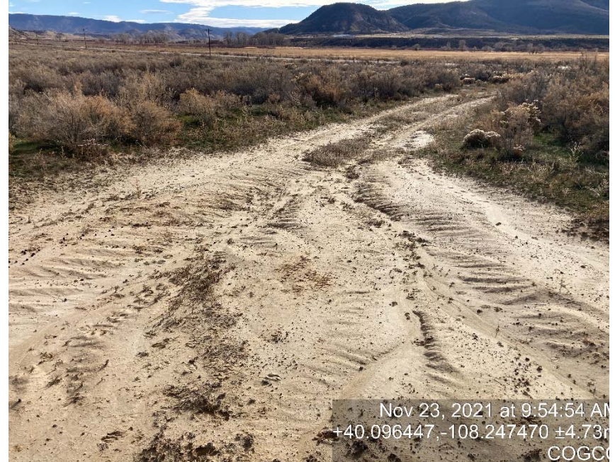
Lack of stabilization/compaction/erosion
