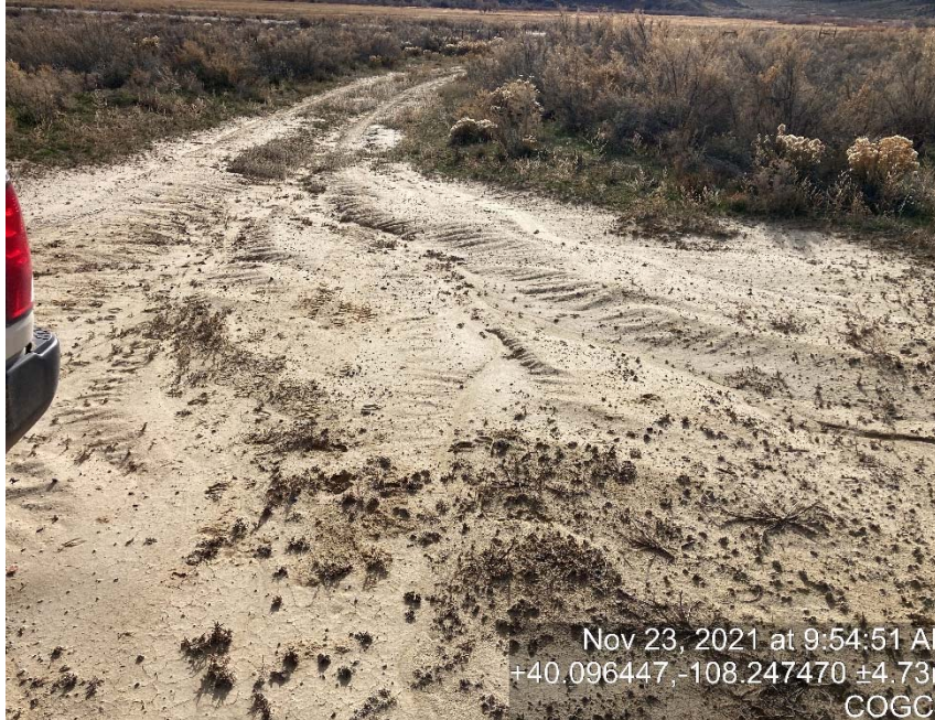
Lack of stabilization/compaction/erosion
